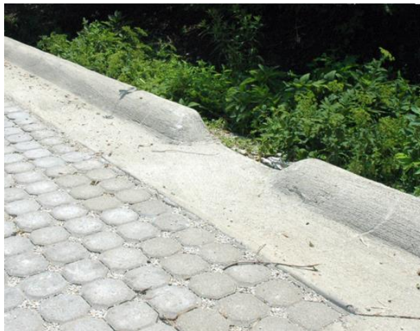
Figure 1119-A: Cuts in the continuous curb allow for stormwater to be directed into landscaped areas.
