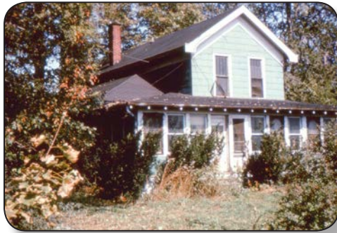
Home on the former Joseph Fitch property demolished to make way for the library
