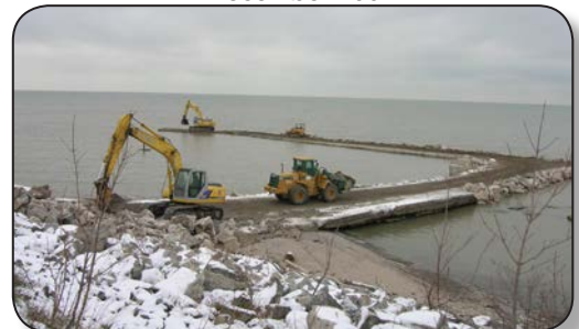
Sheffield Lake Marina under construction, December 2007
