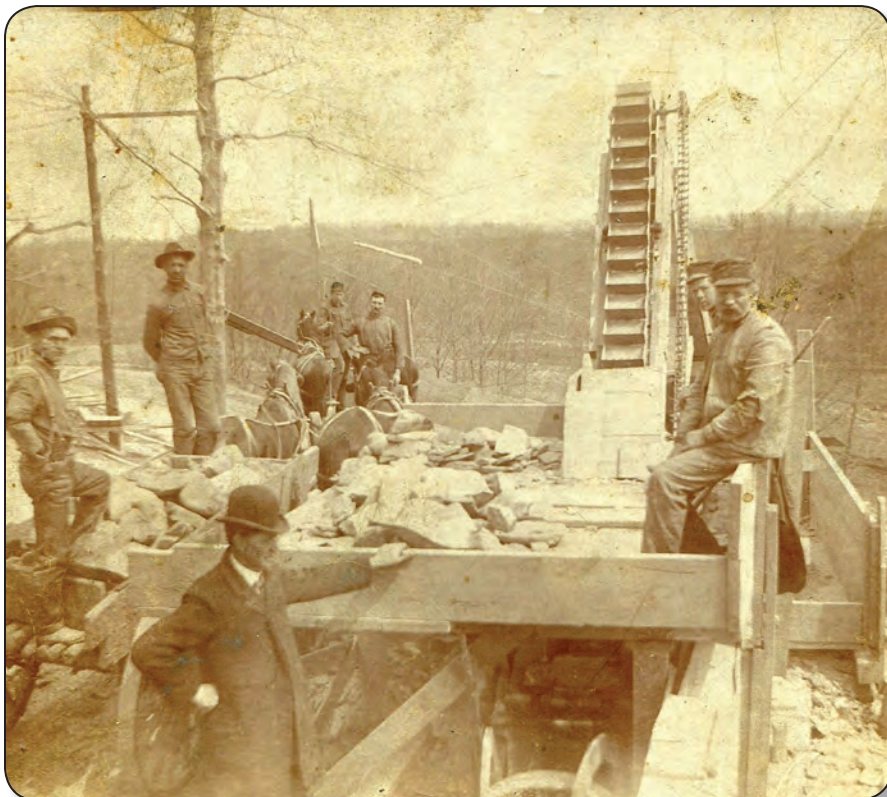
Members of the Herdendorf family working on enlargements of the Erie Canal, circa 1860.
