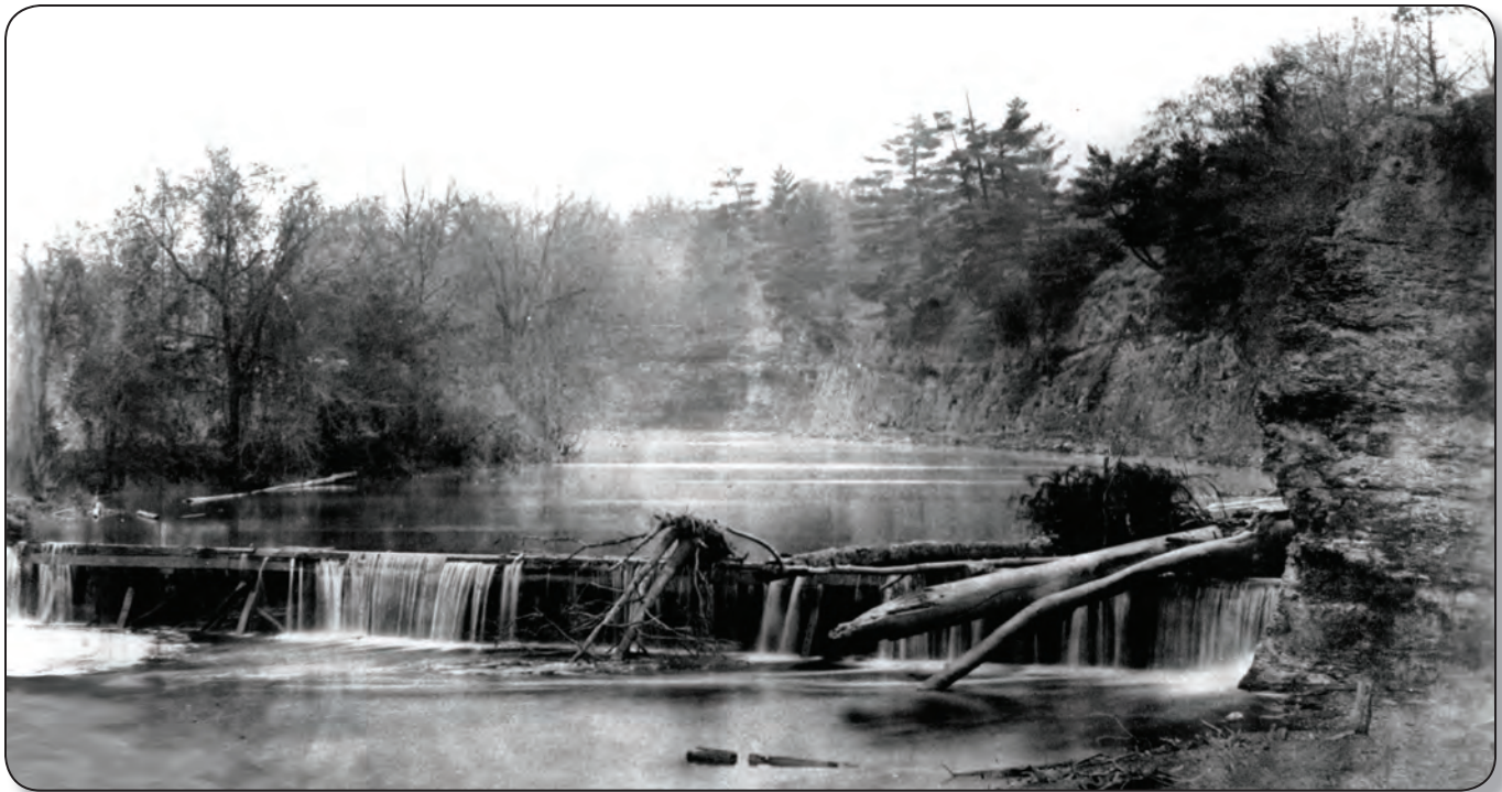
Day's Dam on the Black River, once located upstream of Day's mills to provide a constant head of water for operating the waterwheels (Lorain County Historical Society).
