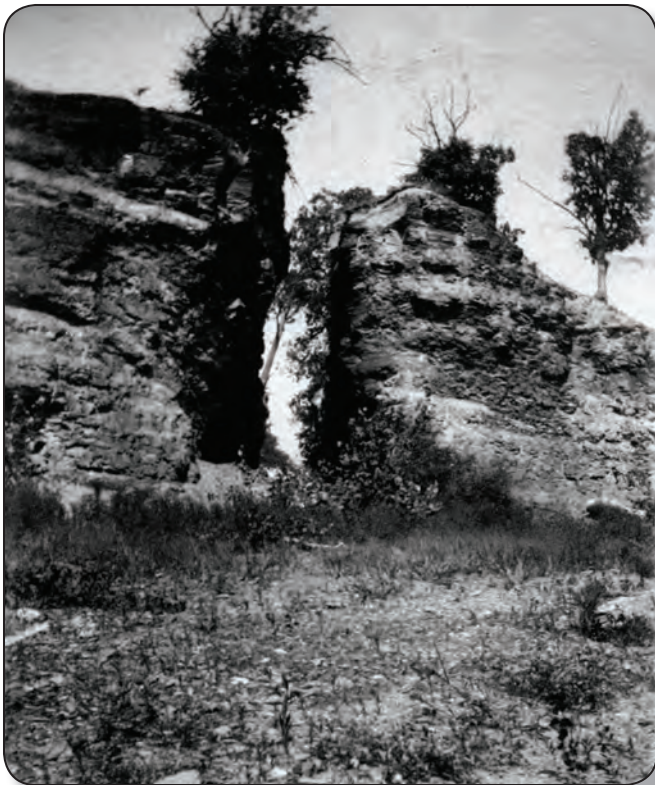
Tunnel cut in the shale bank of the Black River to form a raceway to conduct river water from behind the dam to the waterwheels at the mills (Lorain County Historical Society).
