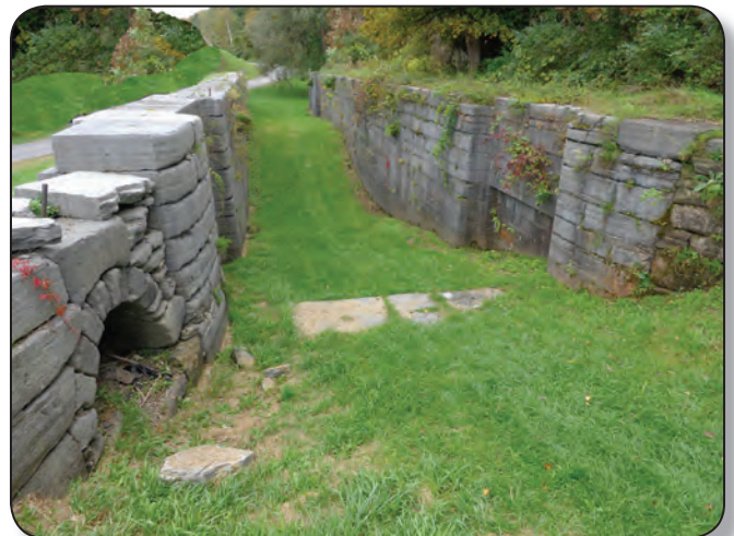
Remains of the canal and locks at Little Falls, New York, which were used by boats to bypass the rapids on the Mohawk River in the early 1800s.
