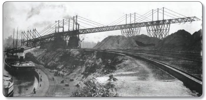
McMyler hoist ore unloader at the steel mill dock on the Black River (circa 1900).
