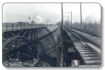
Causeway under construction leading to the steel girders portion of the first East 31<sup>st</sup> Street Bridge in 1913. Photograph taken from Avon Beach & Southern electric railway trestle, built in 1905, toward the east. Note impressive stonework for the causeway's retention wall (Black River Historical Society).
