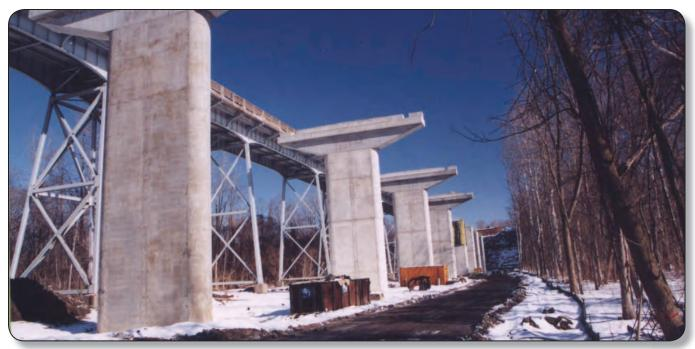
Concrete pillars for construction of new Garfield Bridge in 2000 with original Garfield Bridge in the background (Thomas Hoerrle).
