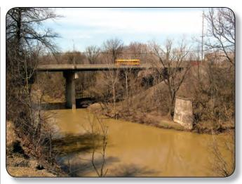
*New East 31st Street Bridge built in 1977 to replace the 1913 structure. Note the abandoned concrete pillar from the 1905 Avon Beach & Southern electric railway trestle.*
