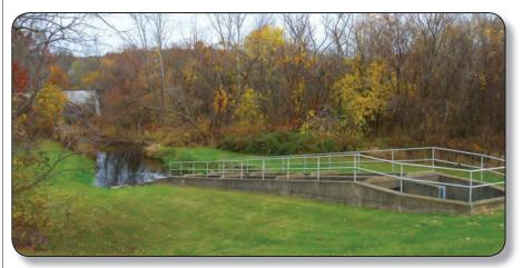
*Outfall structure on French Creek at the end of the treatment process, where up to 5 million gallons of water are discharged to the creek each day.*
