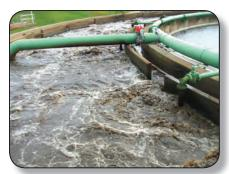
Primary Clarifier Tank where aeration separates sewage and microbes digest the sludge in the outer ring. Sludge is deposited in the quiescent waters of the center ring.
