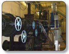
Fourth level down of the Administration Building where the main interceptor pipe enters the plant (left). Pumps (right) lift the wastewater to the Mixing Well where the treatment process begins.
