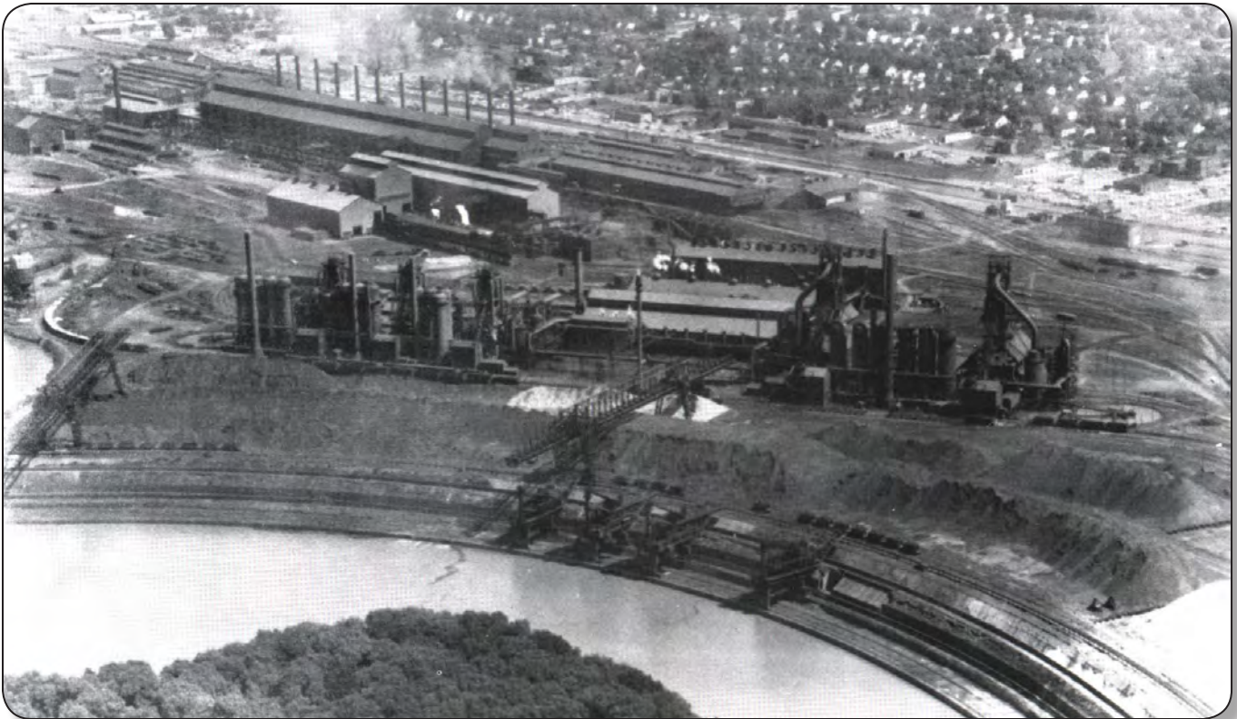
Aerial view of U.S. Steel's National Tube Company on the Black River in Lorain, Ohio, circa 1950; bottom to top, Hulett unloaders, ore bridges/stock yard, blast furnaces, mills, and Lake Terminal roundhouse (Great Lakes Historical Society).
