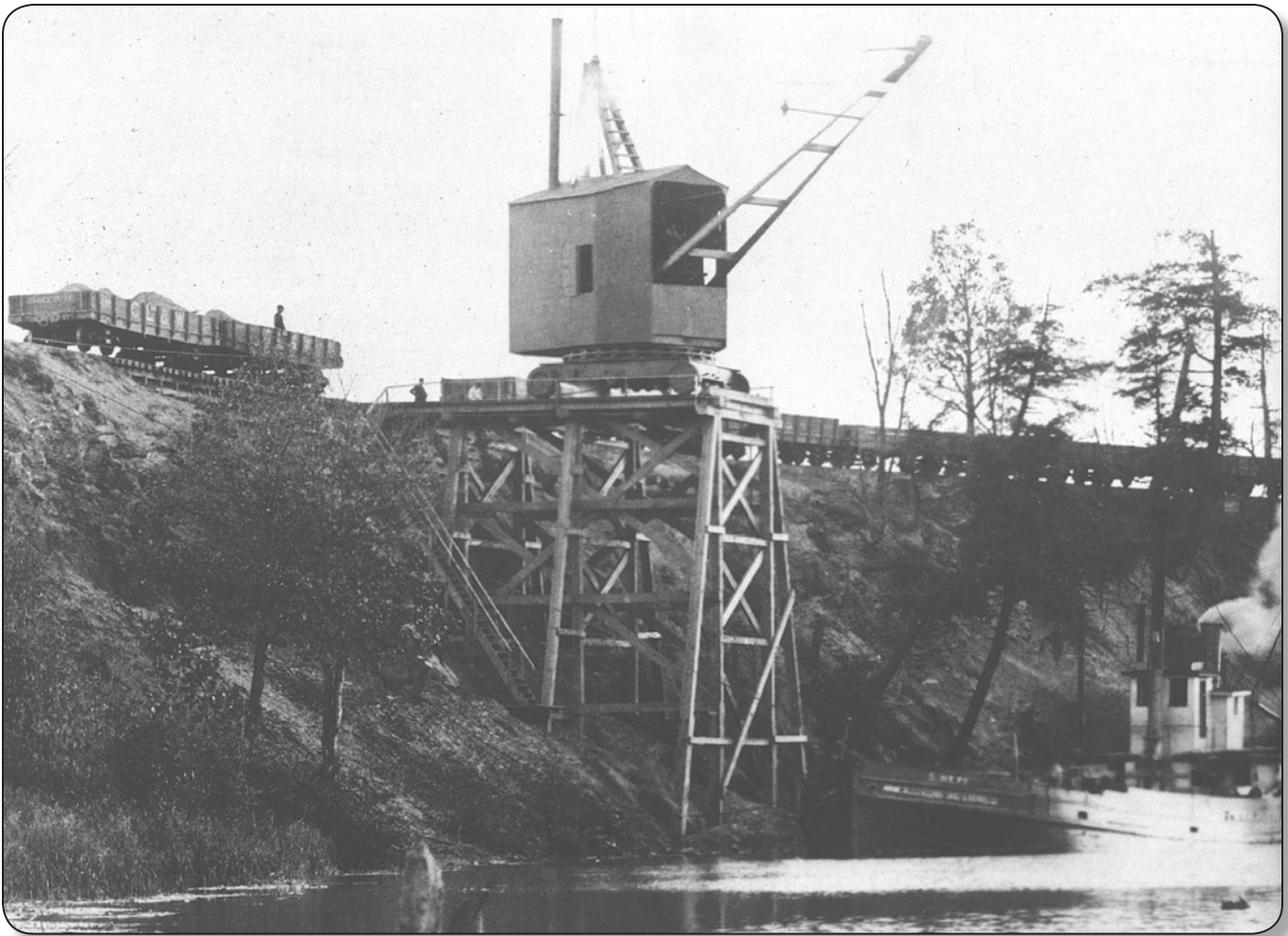
Crane-type ore unloader at the Johnson Steel Company's Black River dock; iron ore is being unloaded from a lake steam barge and loaded into Lake Terminal Railroad gondola cars, circa 1895 (Lorain Historical Society).
