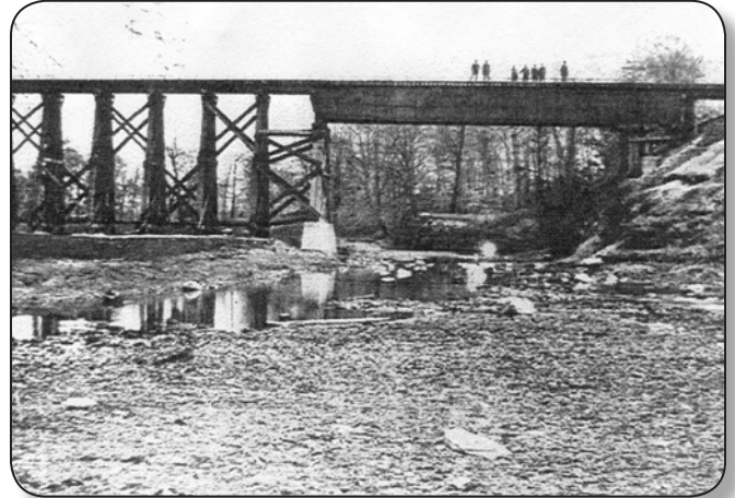
Lake Erie and Pittsburgh Railroad trestle over French Creek in Sheffield, built in 1917 (Lorain County Metro Parks).
