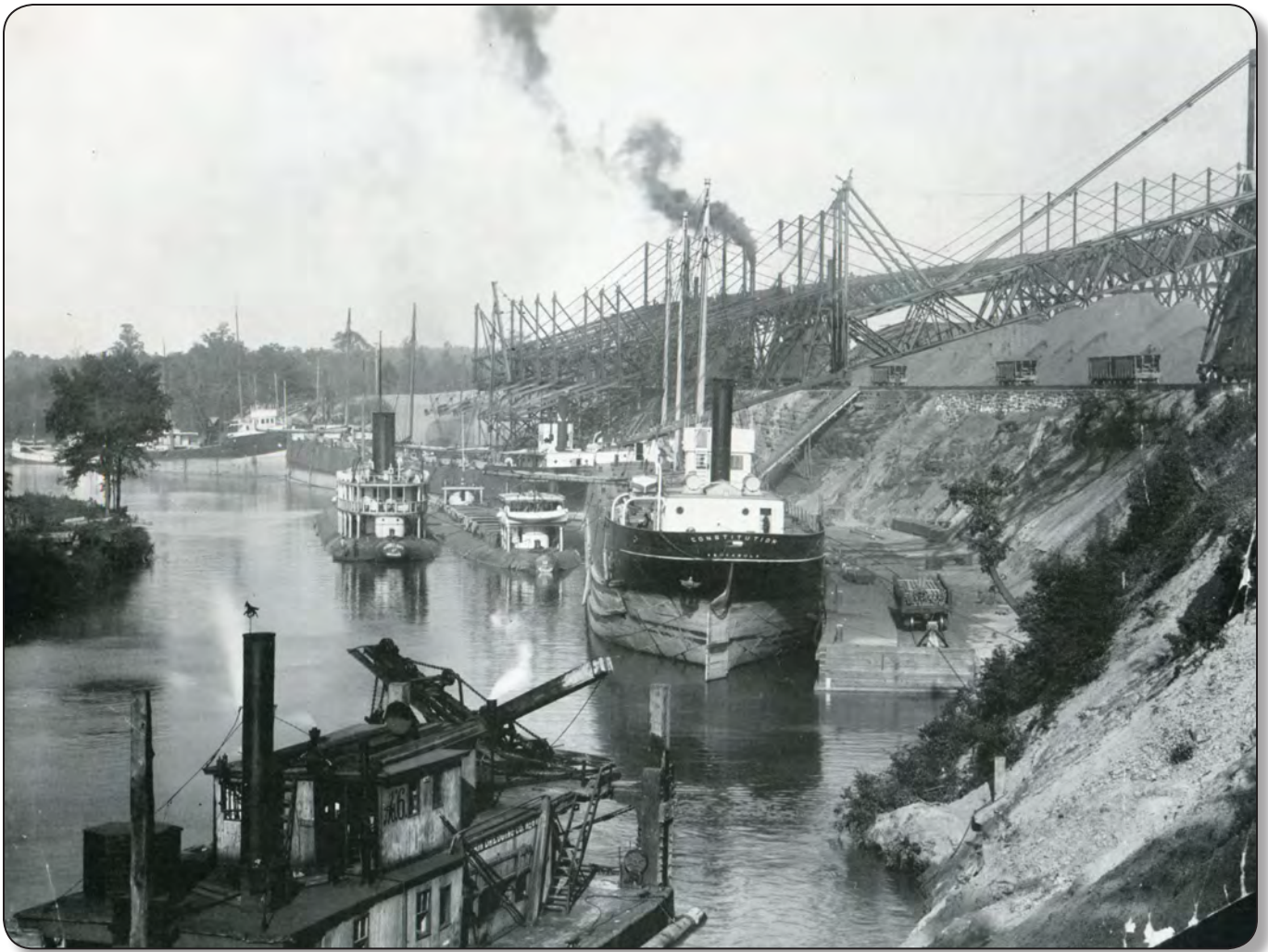
National Tube Company's dock on the Black River; rail-mounted McMyler hoists are transferring ore from freighters to a storage yard at the mill, circa 1899; vessels include the steam barge Constitution (large vessel ahead of dredge) and two whaleback boats (Lorain Historical Society).
