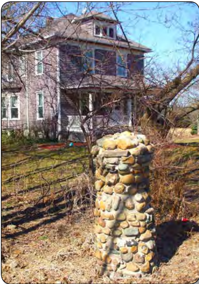
Fieldstone column built by Peter Bungart at 38960 Detroit Road in Avon.
