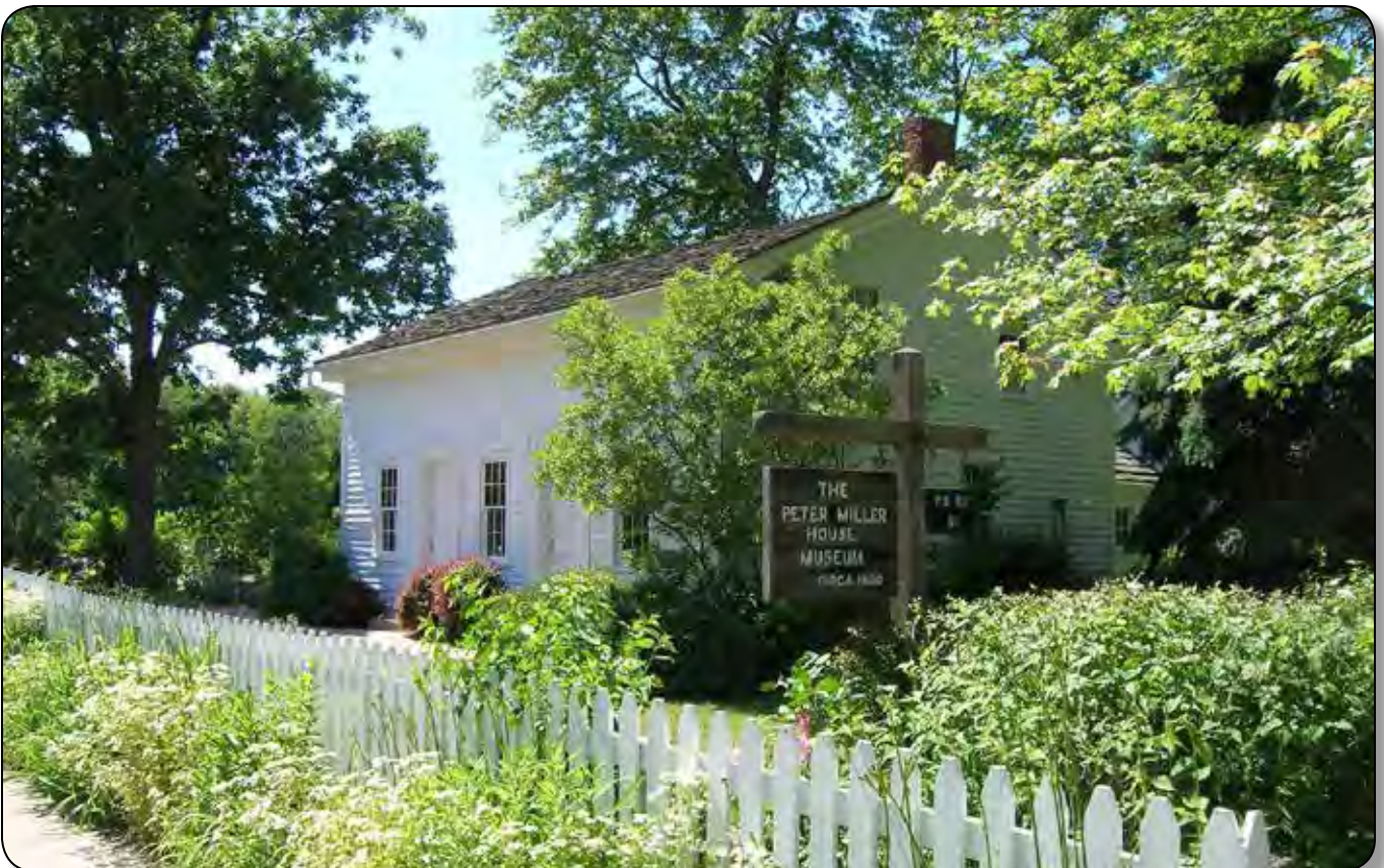
Restored Peter Miller House in Avon Lake, built circa 1830.
