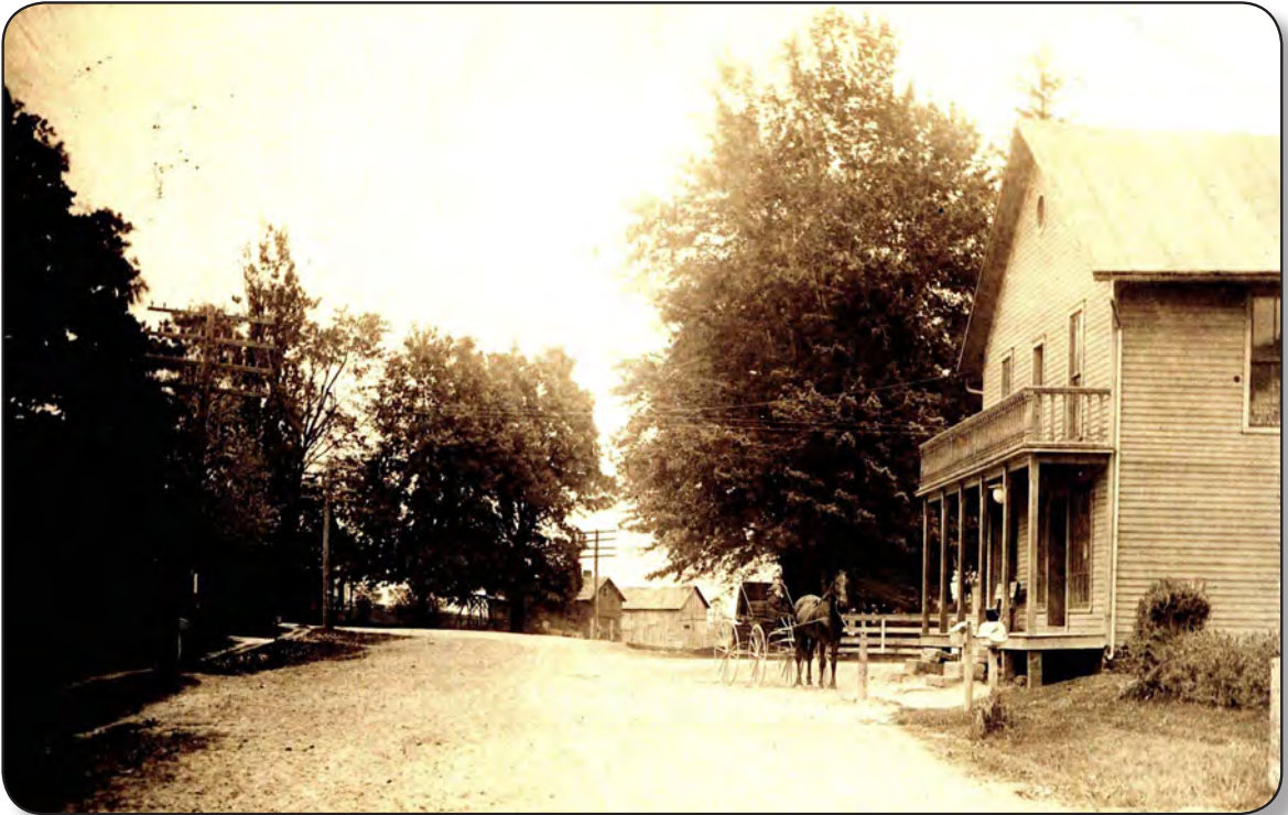
North Ridge at Avon Center circa 1880s (intersection of today's Detroit and Center Roads). Henry Green's Market is on the right. The market sold feed in sacks. Avon women would use the sack material to make dresses. The wooden fence beyond the market encloses Mound Cemetery (courtesy of Avon Historical Society).
