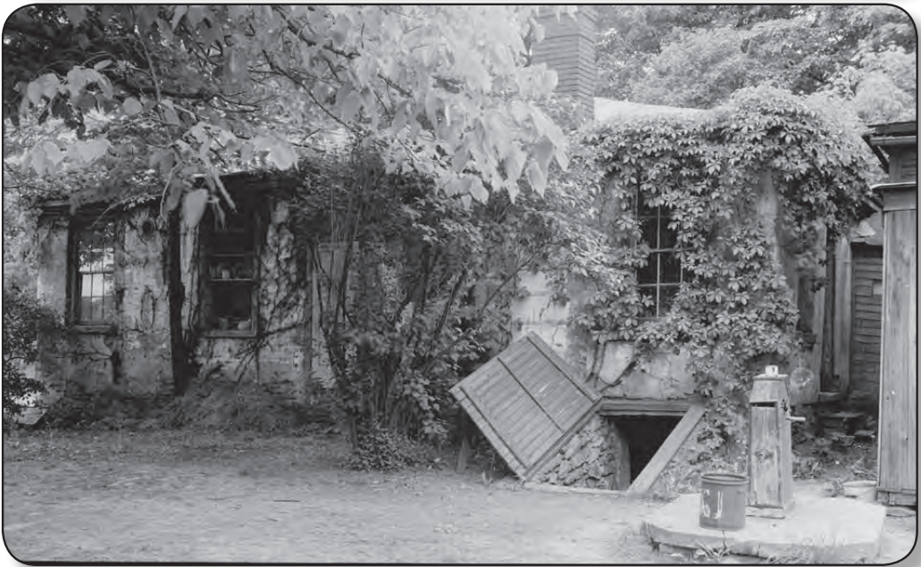
Robinson-Fitch House—Center Road (1936 photographs by Carl Waite, courtesy of U.S. Library of Congress). This house, also known as the Lewis House, is now located in Olde Avon Village—36840 Detroit Road.
