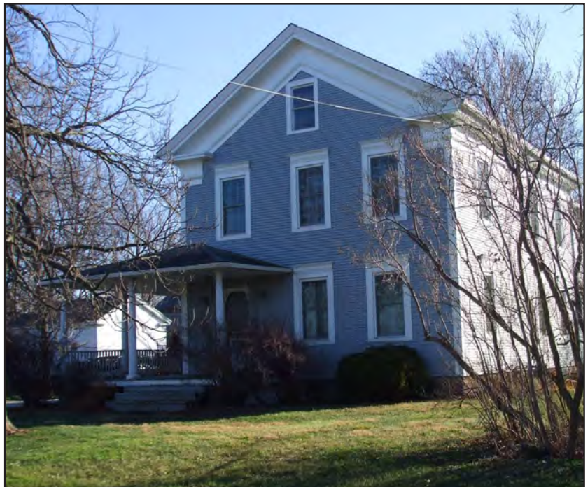
Greek Revival-style farmhouse built circa 1850—33211 Detroit Road.
