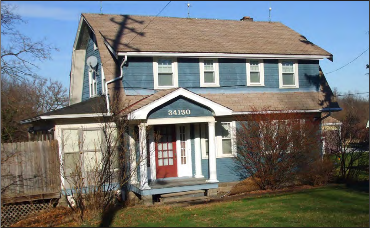
Dutch Colonial Revival-style farmhouse built circa 1900—34130 Detroit Road.
