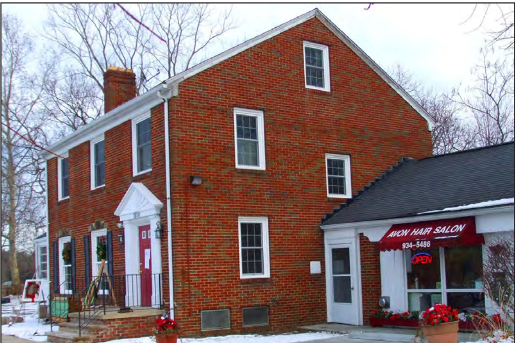
Carriage House, built circa 1945 as a Colonial Revival-style house—36741 Detroit Road.
