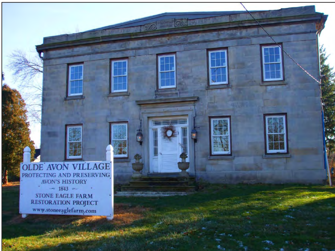
William Hurst House undergoing restoration.
