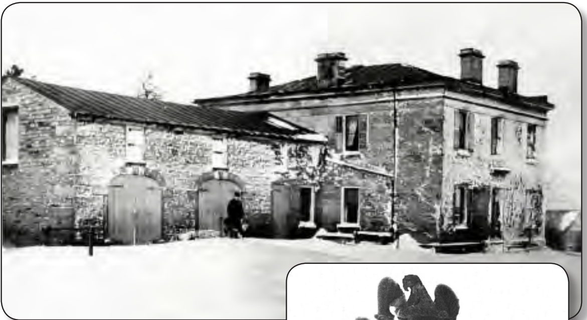
William Hurst House (Greek Revival 1843) at 33065 Detroit Road, Avon, showing service wing built circa 1930s of field stone and sandstone rubble (courtesy Avon Historical Society).
