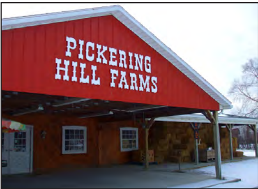
Pickering Hill Farms Market, built 1997.
