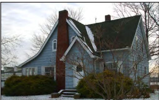
Oebker House— 35651 Detroit Road. This Colonial Revival-style farmhouse, built circa 1920 next to Pickering Hill Farms, shows elements of Tudor Revival style especially in its steeped-pitched roof, front gable entrance vestibule, and full-height masonry chimney.
