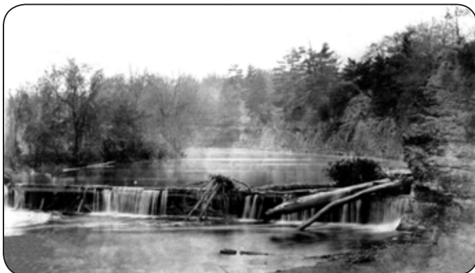
Day's Dam was located on the Black River a short distance upstream from Day's Mills. The dam supplied a constant head of water to operate the waterwheels at the mills (Lorain County Historical Society).
