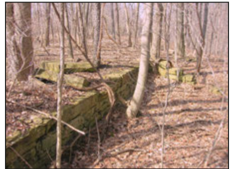
Foundation remains of the 1880 schoolhouse at Sheffield Center.
