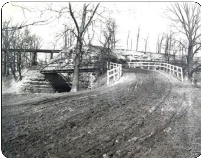
Day's Dam Bridge over the Black River was located a short distance downstream from Day's Mills before the East 31 st Street Bridge was constructed in 1913 (Albert Doane).
