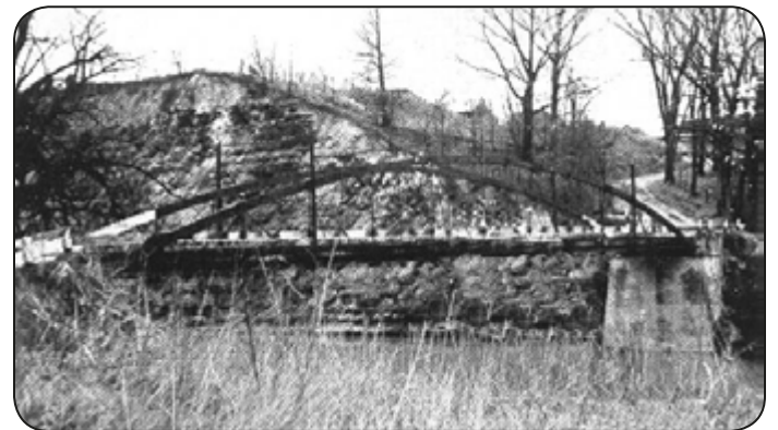
North Ridge Bridge over the Black River at the bottom of Gashouse Hill. This steel-truss bridge served until Garfield Bridge was constructed in 1936 (Ohio Department of Transportation).
