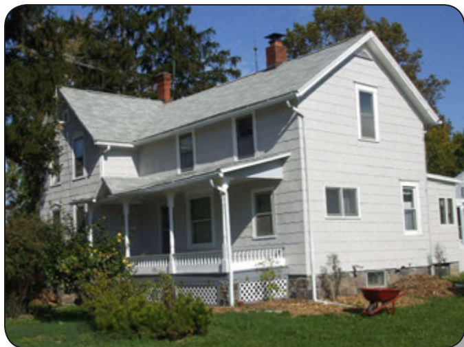
Ackerman Family farmhouse built in the 1860s, exterior restoration completed by the family in 2008.
