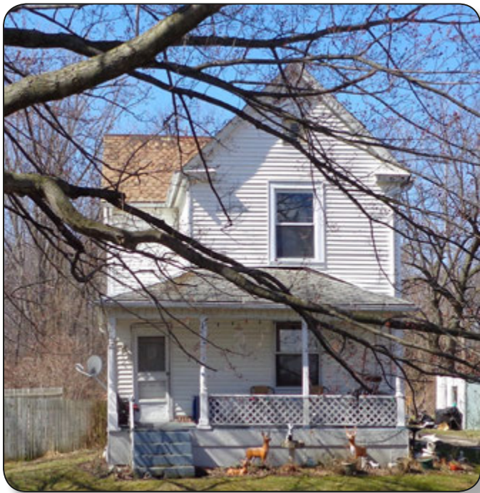
John Fox House at 998 Lake Breeze Road in Sheffield Lake (built c1840).
