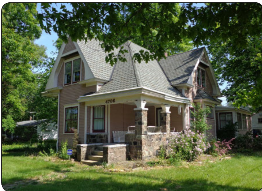
John Ferner (1881-1971) House at 4706 Lake Road in Sheffield Lake (built 1906).
