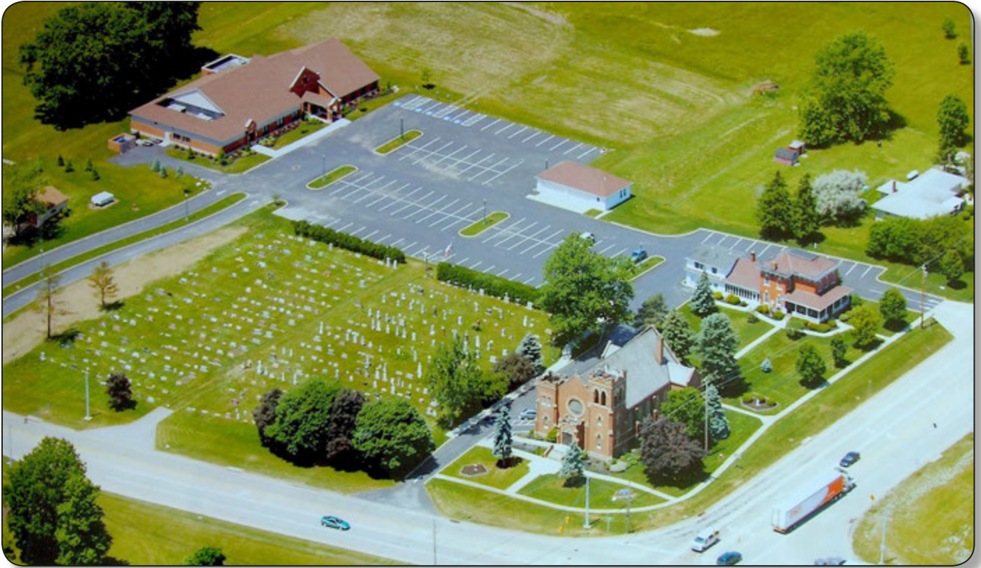
Aerial View of Saint Teresa of Avila Parish Grounds.
