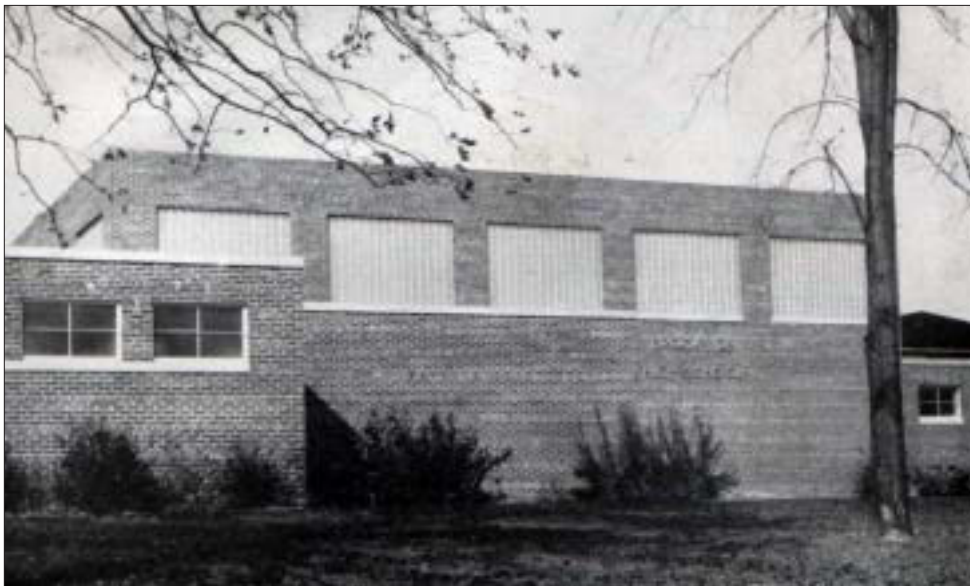
Brookside High School's gymnasium wing constructed in 1955 (courtesy of The Leader).
