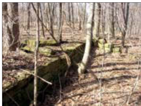
Foundation of District No. 1 Schoolhouse (2007).
