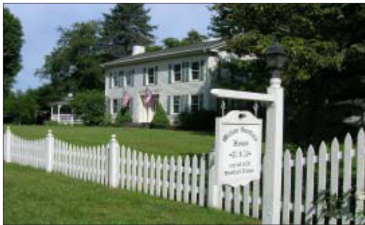
Milton Garfield House (1839).
