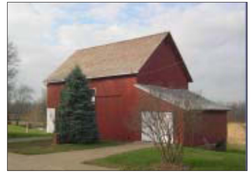
Daniel Garfield Barn at 5013 Detroit Road before it was taken down in 2005.
