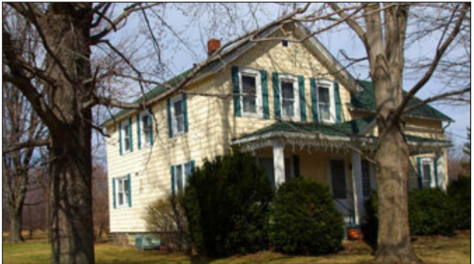
Kelling House (5351 Colorado Avenue).
