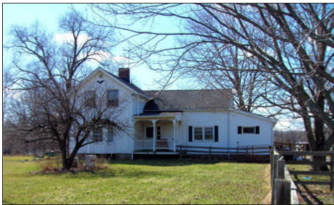
Forster/Schuëller House (1736 Abbe Road).
