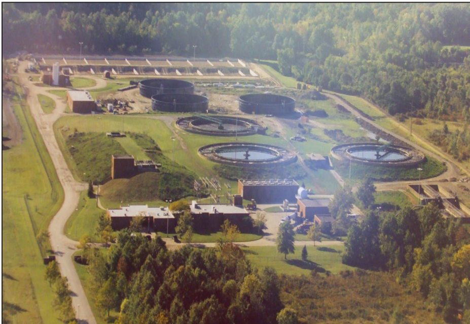
Aerial view of French Creek Wastewater Treatment Plant in 1996. Administration Building at lower left, Grit Building at center left, Sludge Building at upper left, and clarifier tanks at center right (courtesy of the City of North Ridgeville).
