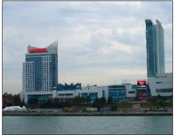
Windsor's Caesars Casino from the Detroit River.
