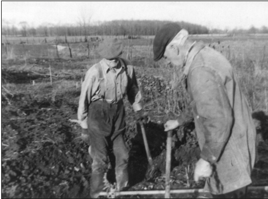
John Emerick (right) and Harry Root installing a drainage tile between their farms, circa 1954.
