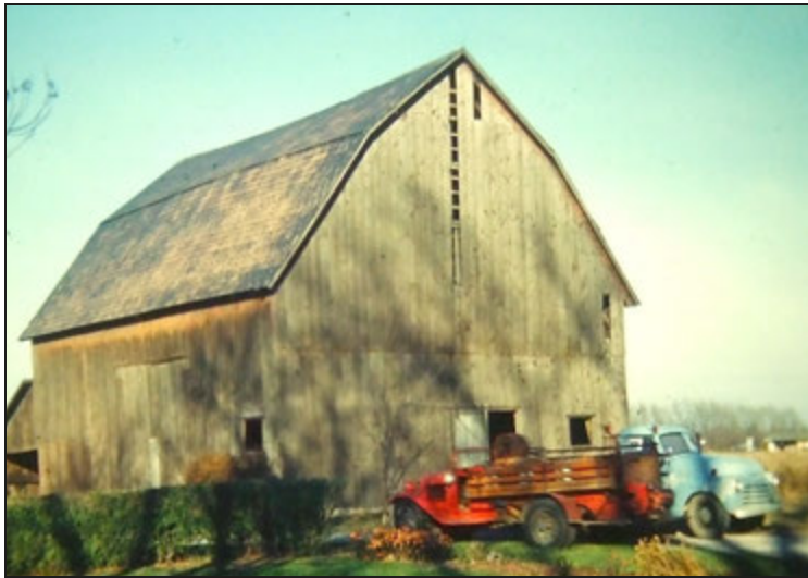
Barn on Lake Breeze Road being prepared for a practice fire.
