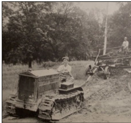
Models K-20 and A-30 Cletrac tractors were successfully used on farms (a) and for road grading (b) in the United States and Europe in the 1920s–1940s (courtesy of Mike Stockard).
