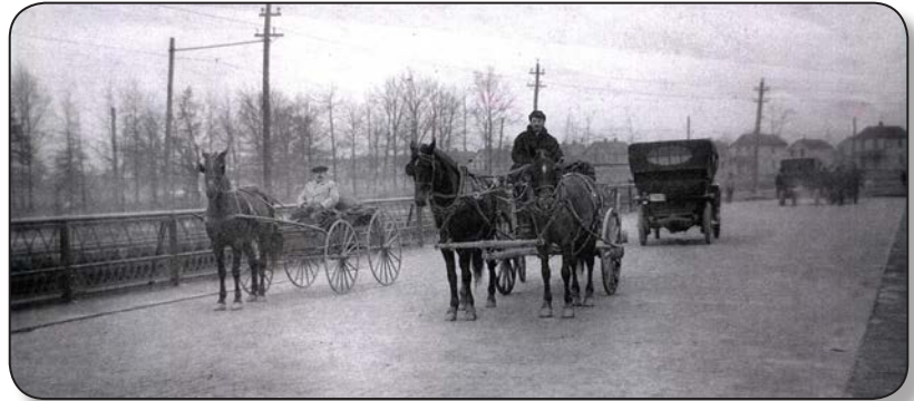
Early traffic on 1913 East 31 st Street Bridge
