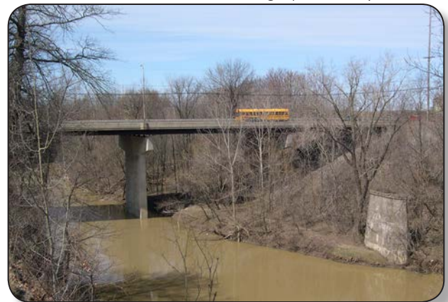
New East 31 st Street Bridge (built 1977)
