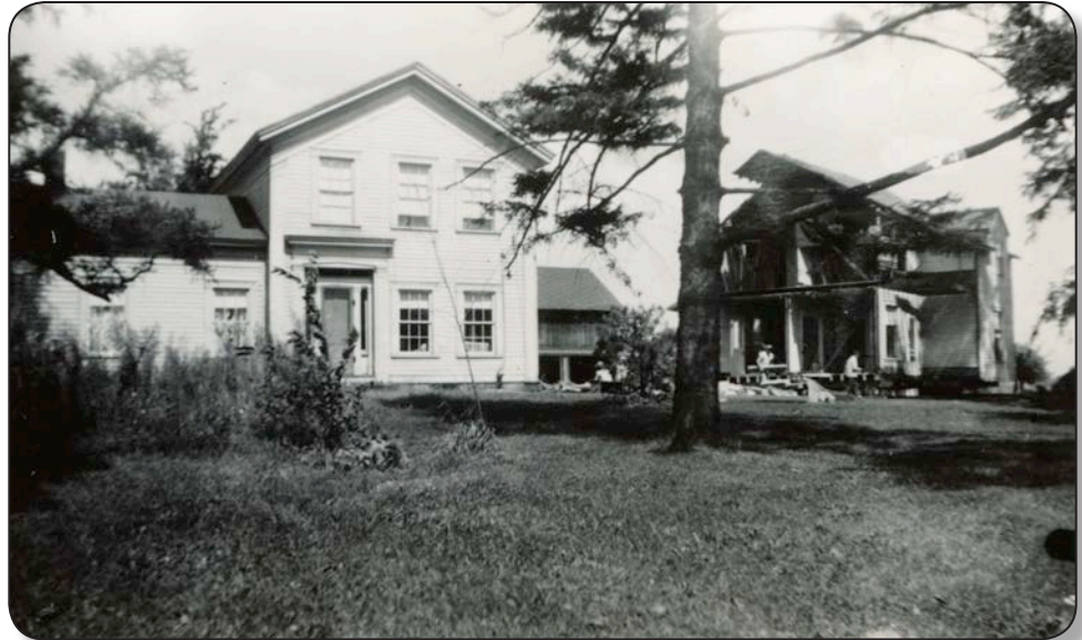
Halsey Garfield House in the process of being split into two dwellings on the late 1930s
