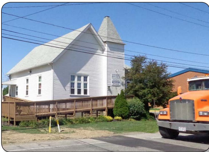
Faith House Day Care Center adjacent to Vincent School (2014)
