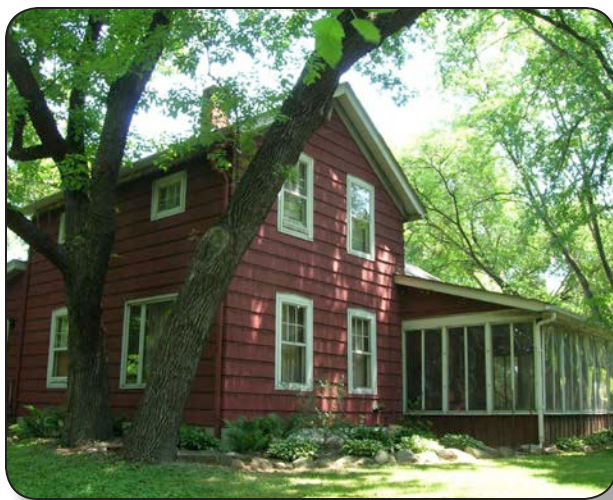
Front of Bedortha-Traxler House that originally faced Old Colorado Road
