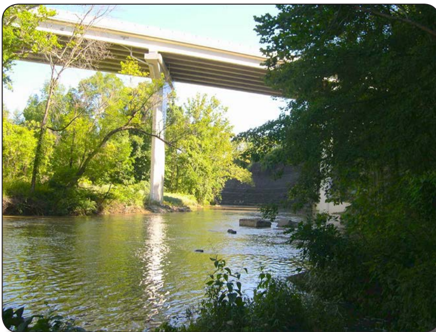
New viaduct bridge, 2003
