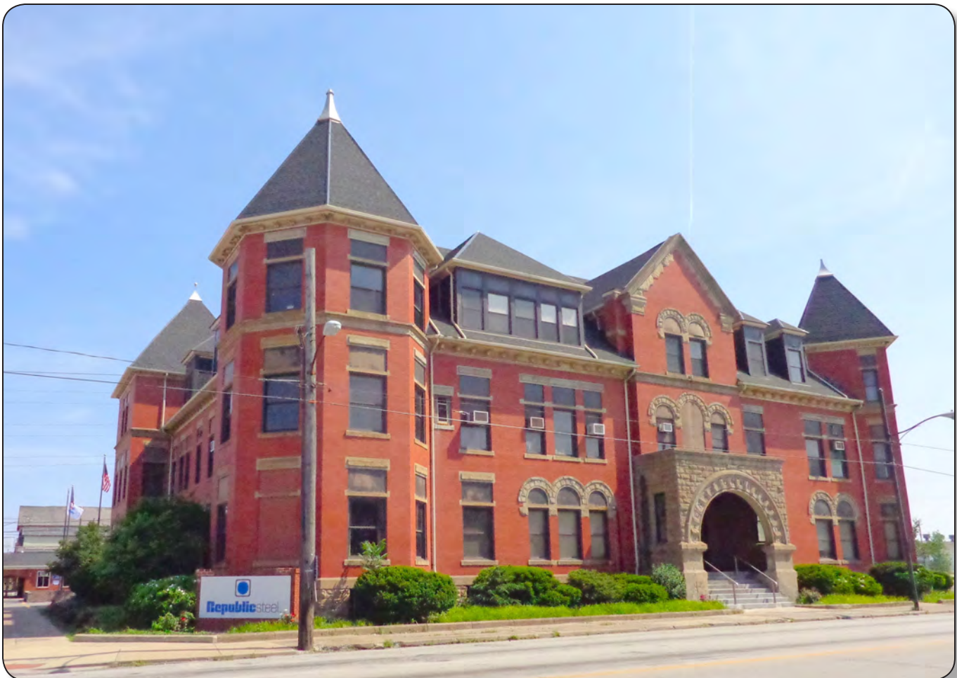
Johnson Steel Company Office Building erected in 1895 on land that was originally in Sheffield Township. This building on East 28 th Street now serves as headquarters for Republic Steel Corporation’s Lorain mills. This structure is on the National Register of Historic Places.
