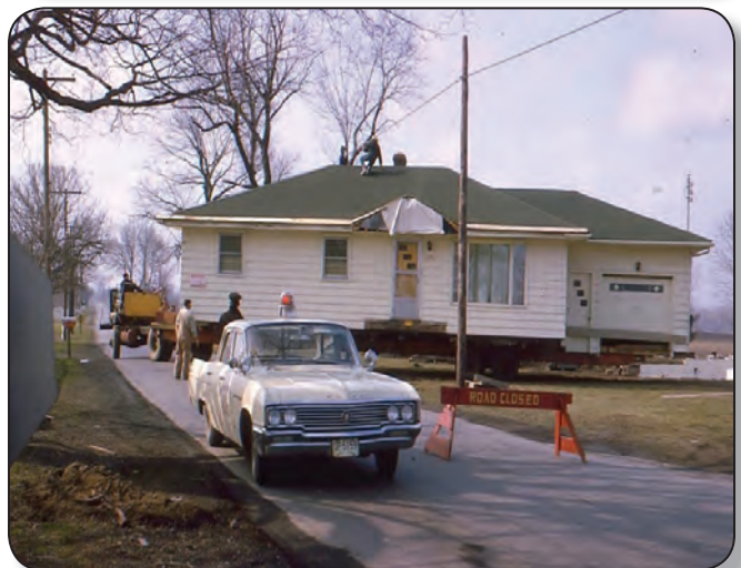
Chuck Gubeno's house at southwest corner of intersection being moved farther south on Abbe Road when Detroit Road was widened. This house was later torn down to make way for the Cobblestone shopping area.
