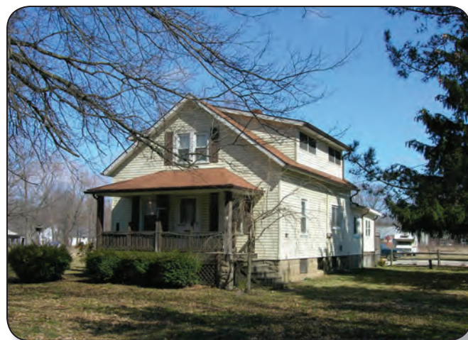
The Ferguson House at 4567 East River Road in 2007, now the home of the Dennis German family.
