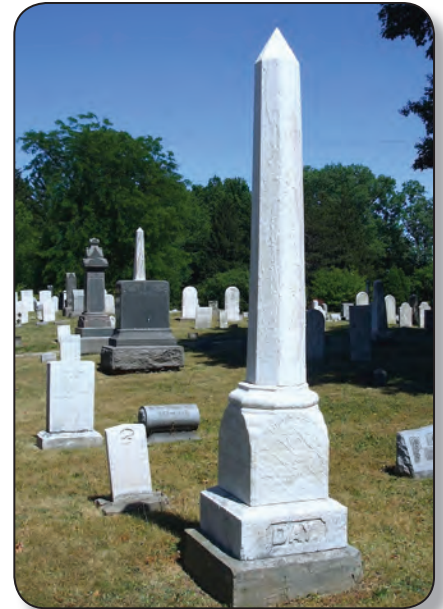
John Day monument shines after treatment with enzyme cleaner and heated power wash.
