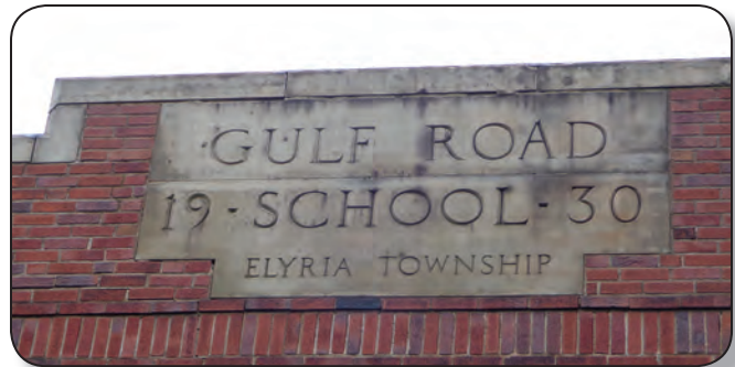
Gulf Road School, Elyria Township, built in 1930.
