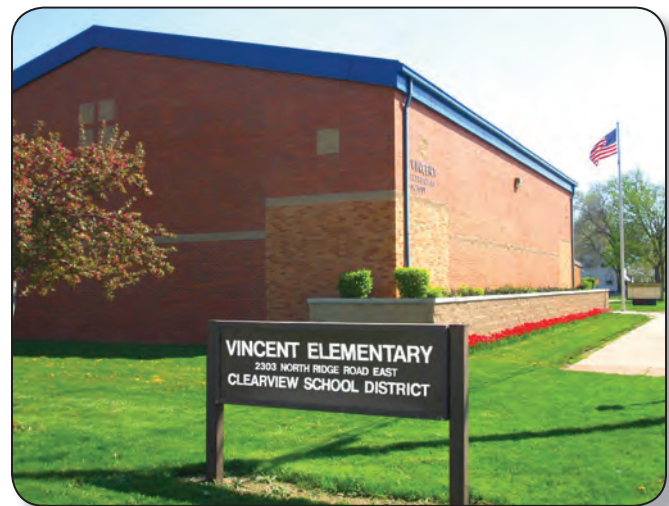
Vincent Elementary School (2014).
