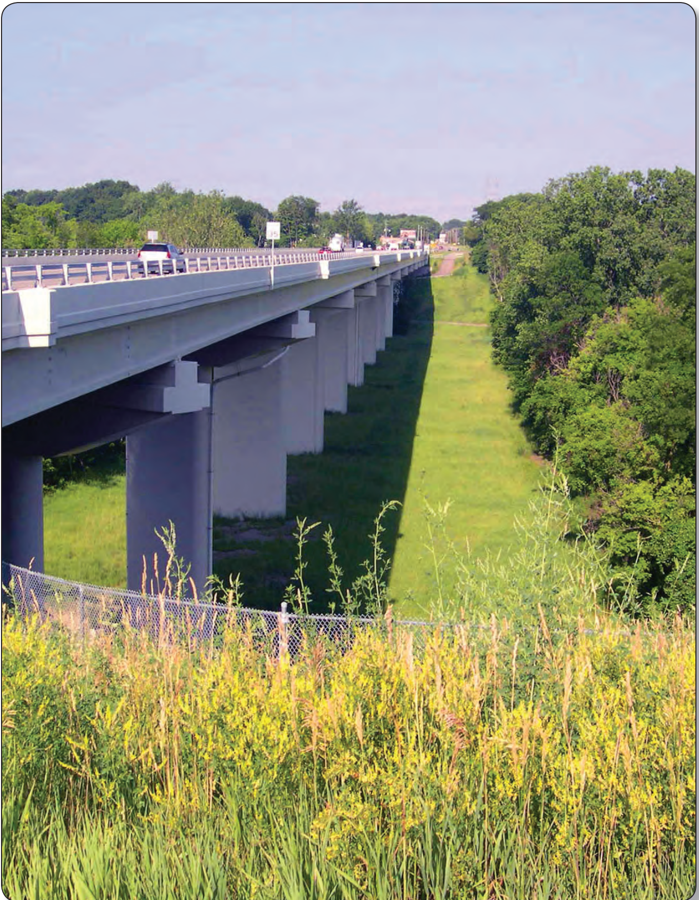
New Garfield Bridge over the Black River, completed in 2003.
