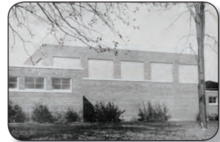
Brookside High School's new gymnasium built in 1955.
