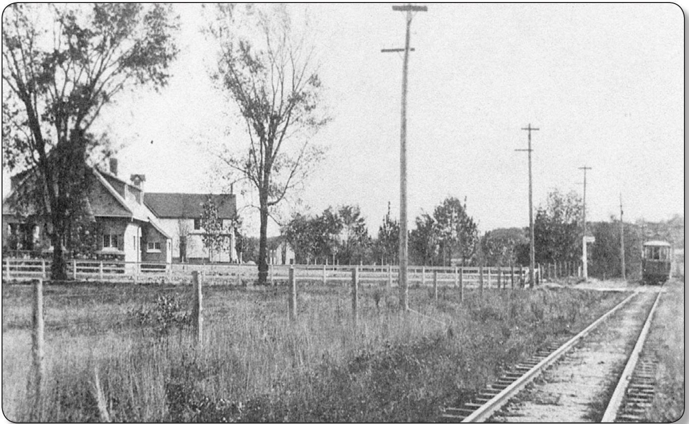
Lorain & Cleveland Railway's high-speed (sustained 50-plus mph), single-track route along Sheffield Township's lakeshore, circa 1900; later acquired by the Lake Shore Electric Railway, a double-track route was constructed in 1906 (John Rehor).
