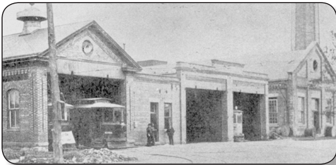
Lorain Street Railway’s South Lorain streetcar barns (left) and power plant (right), built by Tom Johnson in 1894 on 28 th Street at foot of Seneca Avenue; note the notches above the door openings to accommodate the trolley wheels (Albert C. Doane).
