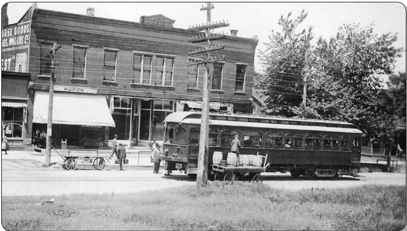
Lake Shore Electric Railway trolley at a storefront depot (Station No. 88) in Huron, Ohio, circa 1910. Used primarily for passenger service, but because the interurban tracks often used downtown streets trolleys did carry some commercial cargo (Willis Leiter).
