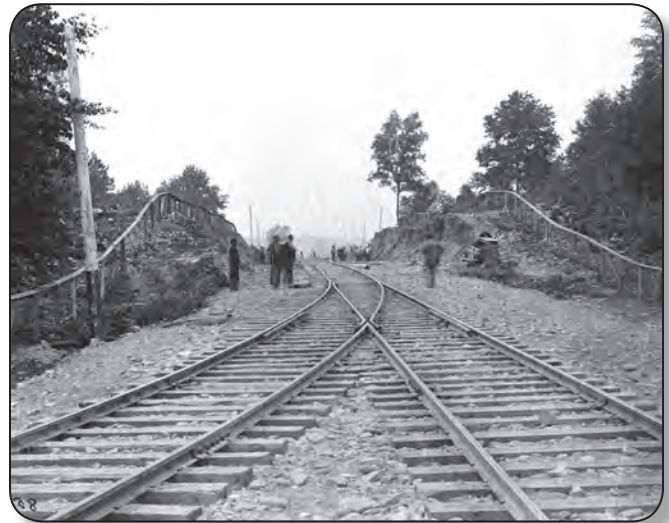
Eschruth quarry siding. As the demand for sandstone foundation material increased during the construction of the Johnson Steel Company and associated housing for mill workers in South Lorain, in 1894 a railroad spur was built to connect the quarry with the main track running between South Lorain and Elyria (Albert C. Doane).
