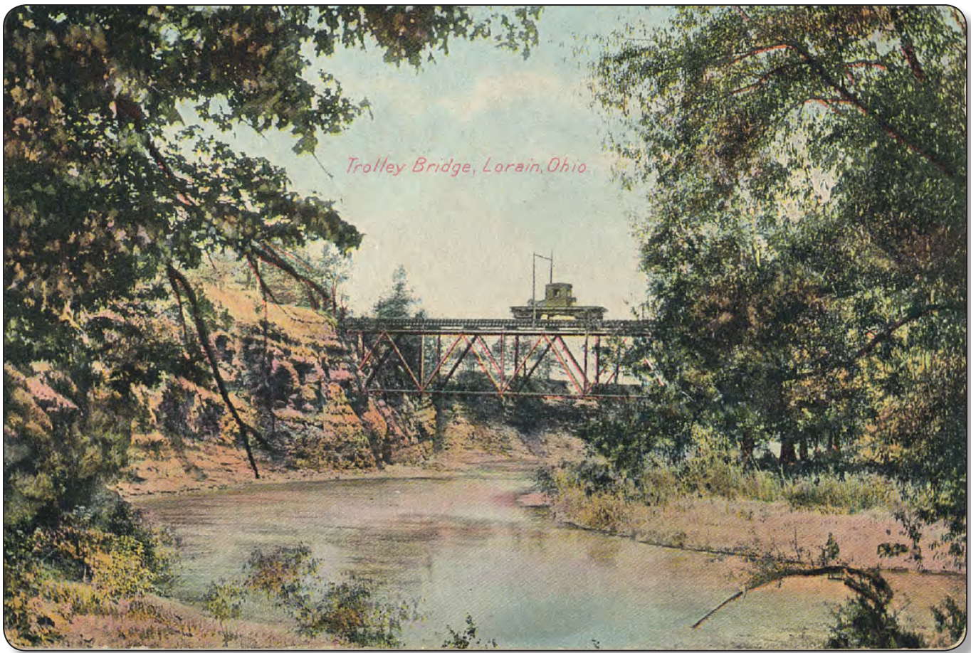
Postcard of a work engine crossing the Avon Beach and Southern electric railway trestle over the Black River, circa 1905. The trestle was located just upstream (south) of the current 31 st Street bridge (Garfield Farms Landmark Foundation).
