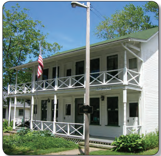
Elfordilno, originally a barracks, now serves as the 103 rd O.V.I. Regimental Museum.
