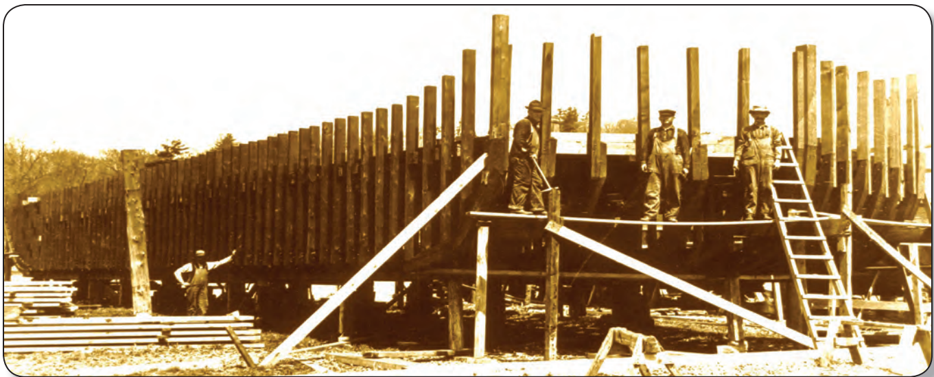
In anticipation of Perry's victory, General Harrison ordered the construction of 80 scows at Cleveland, Ohio to transport 4,500 troops and artillery for an amphibious invasion of Canada near Amherstburg. Commodore Perry used the American fleet and captured British vessels to tow the scows (photograph of scows similar to those used for the invasion, Patrick Labadie).
