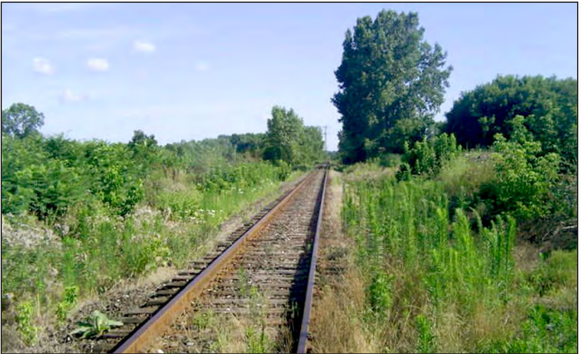
Former Lake Shore & Michigan Southern Railroad tracks, built circa 1890, form the boundary between Sheffield and Avon (photograph by Thomas Hoerrle).
