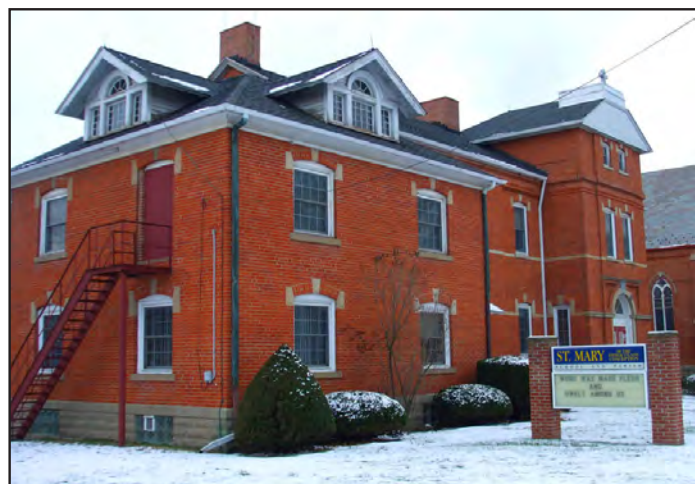
St. Mary School, built 1885—2680 Stoney Ridge Road.
