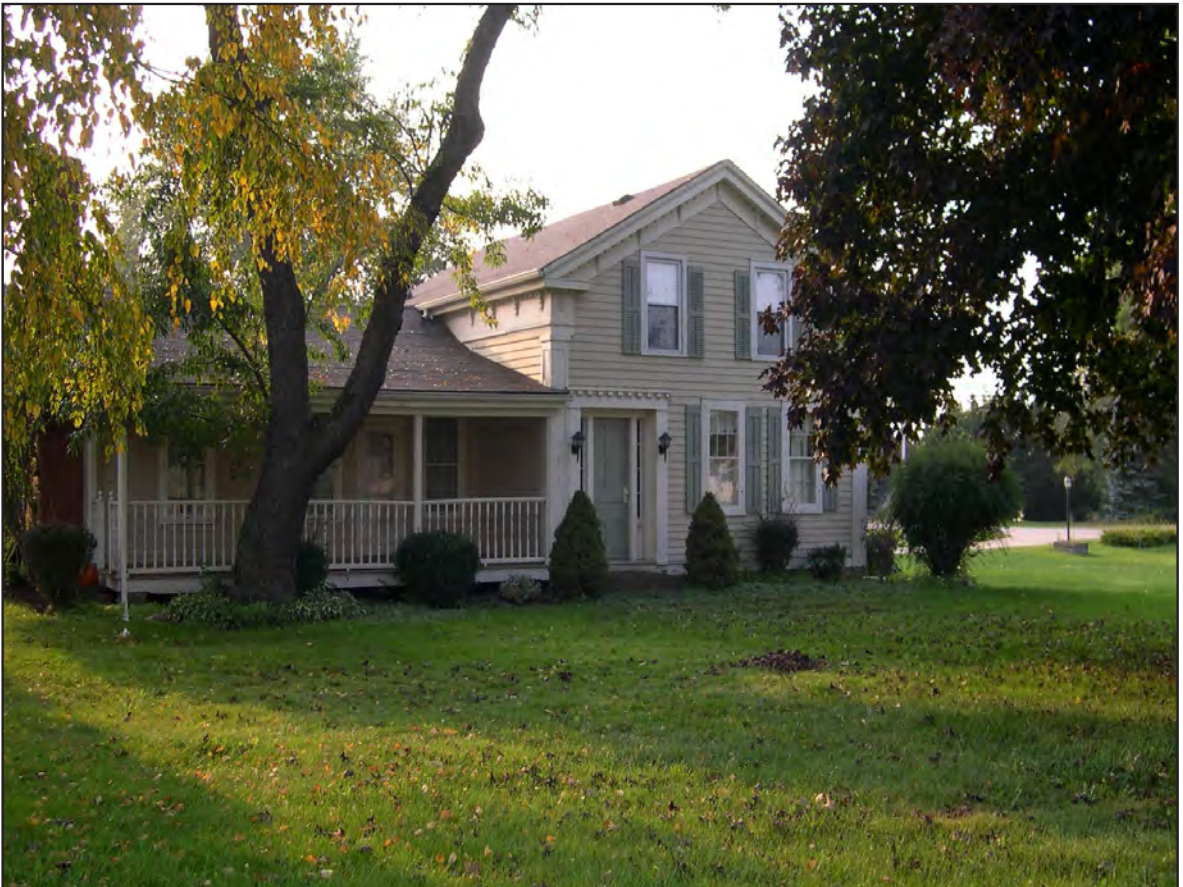
Ezra Jackson House, Greek Revival-style home built by the owner in 1846—39351 Detroit Road.
