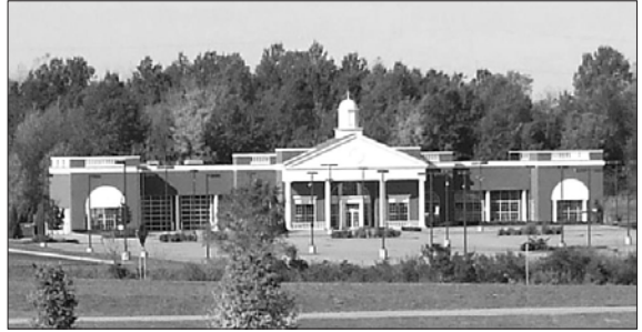
Spitzer Building—4850 Transportation Drive.
