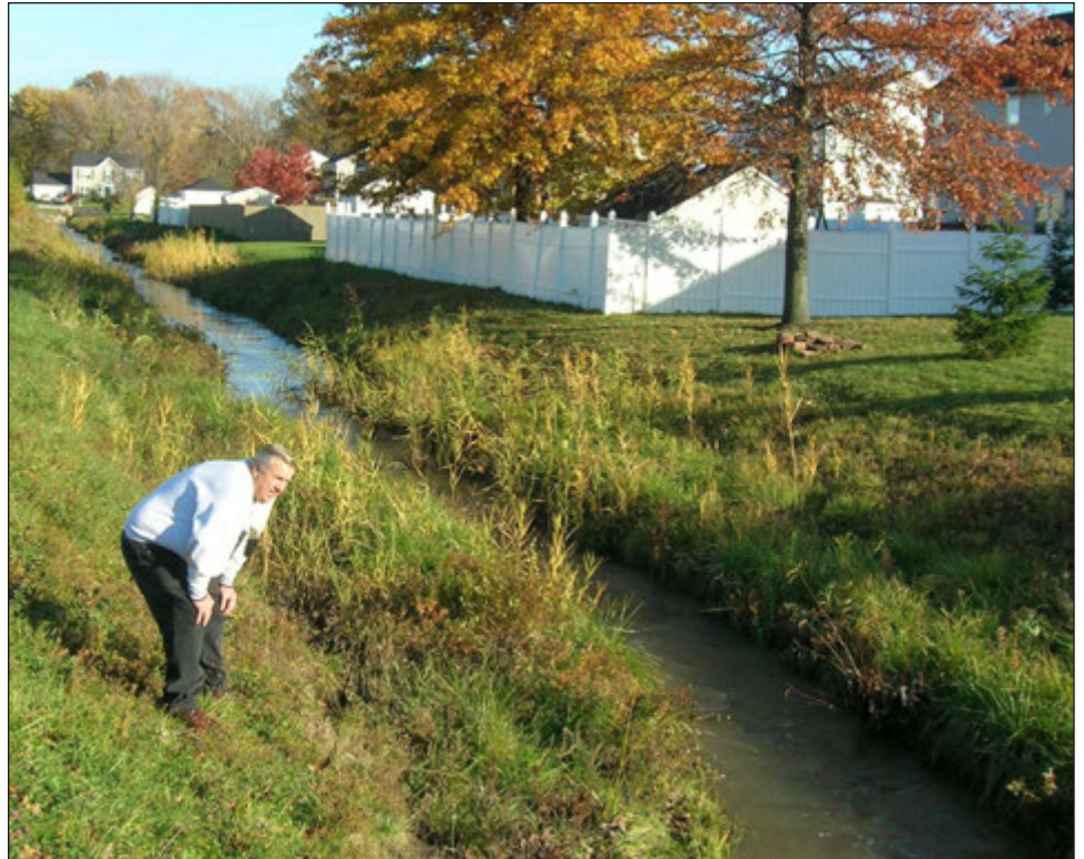
Mayor-elect John Hunter inspects Jungbluth Ditch in College Heights—November 13, 2007.
