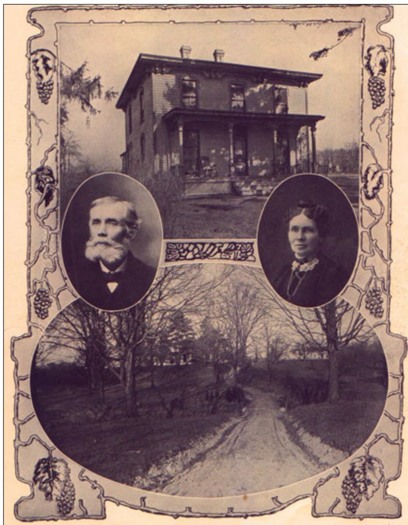
Home of William Augustus Day (1835-1910) and Mary (Steele) Day (1840-1925) on East River Road, built in 1879 (from Lorain County: Picturesque & Industrial Features, 1906).
