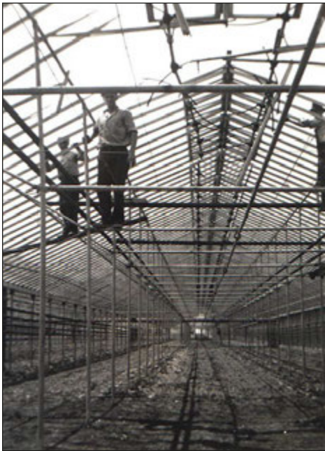
Construction of Hoag's Greenhouses in 1937 (courtesy of Bob and Marilou Hiltabiddle).
