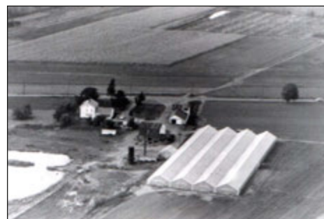
Aerial view of DeChant Greenhouses on Detroit Road in the 1950s (courtesy of Bob and Marilou Hiltabiddle).
