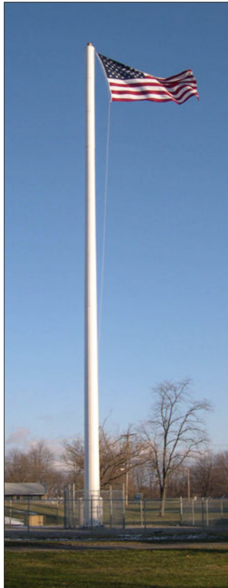
T-Mobile Antenna Tower at the intersection of Gulf and Detroit Roads.
