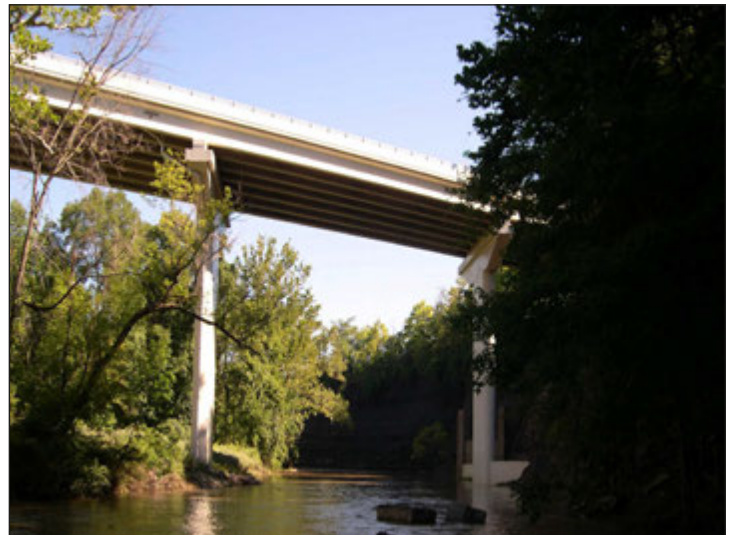
New Garfield Bridge over the Black River from river level in 2005.
