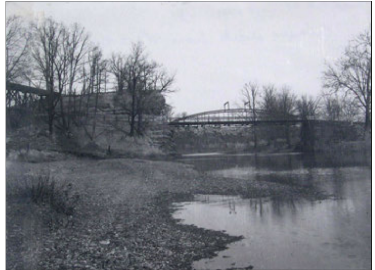
Profile view of Days Dam steel-truss bridge (~1910) over the Black River. Avon Beach & Southern electric railway trestle at far left side of photograph (courtesy of Black River Historical Society).
