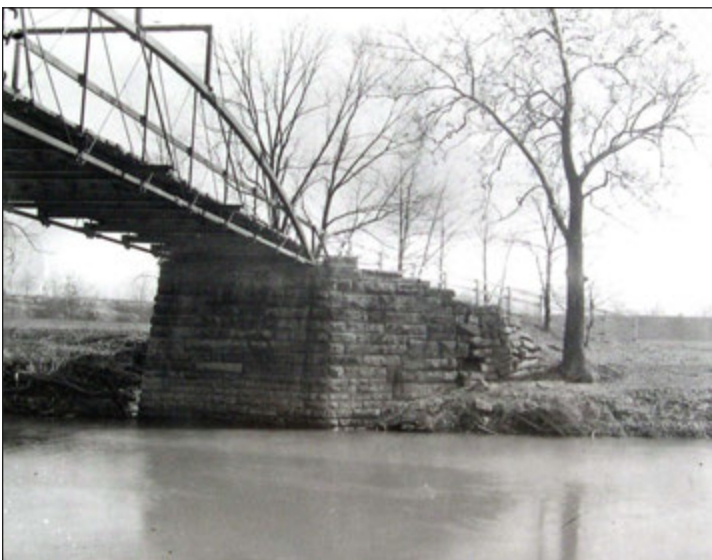
South abutment to Days Dam steel-truss bridge (~1910). The Black River flows under the bridge here, but has since abandoned this meander channel (courtesy of Black River Historical Society).
