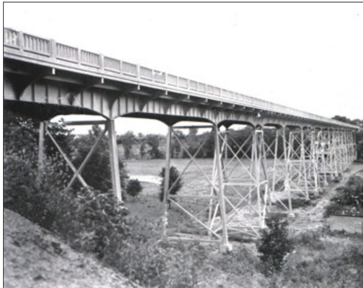
First Garfield Bridge viaduct (SR 254) over the Black River, built in 1936 (courtesy of Ohio Department of Transportation).
