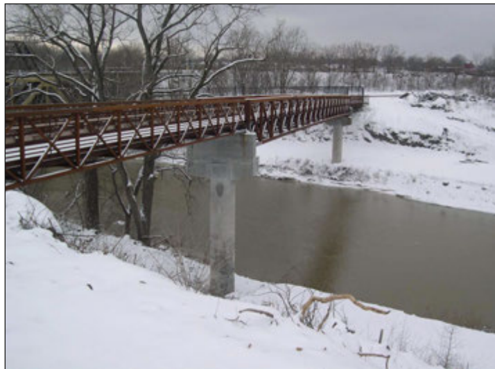
Lorain County Metro Parks' new 40-foot-high Steel Mill Trail bridge over the Black River about one-quarter-mile downstream of the East 31 st Street bridge.
