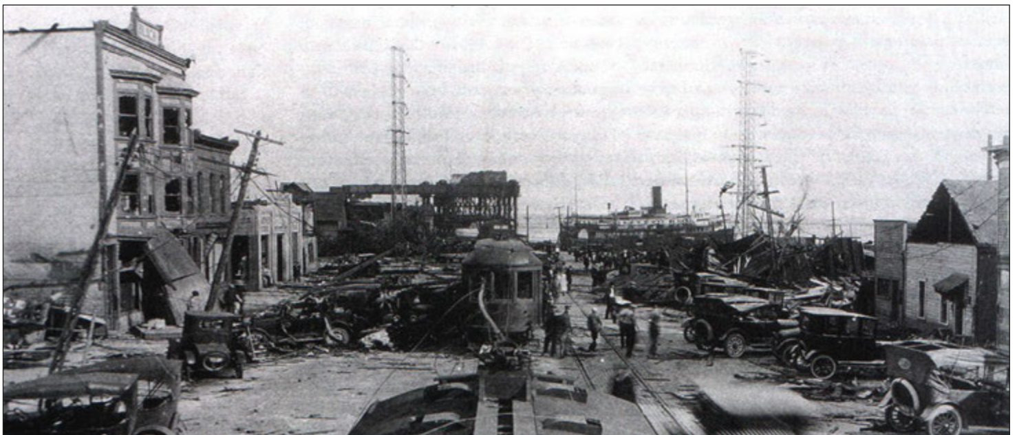
Destruction of downtown Lorain by June 28, 1924 tornado, showing damaged power lines and disabled trolley cars (courtesy of Albert C. Doane).
