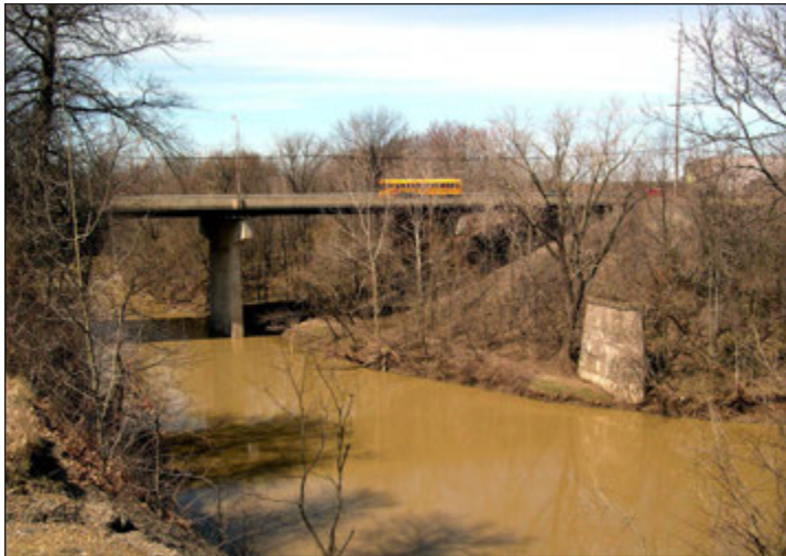
New East 31 st Street Bridge built in 1977 to replace the 1913 structure. Note the abandoned concrete pillar from the 1905 Avon Beach & Southern electric railway trestle.
