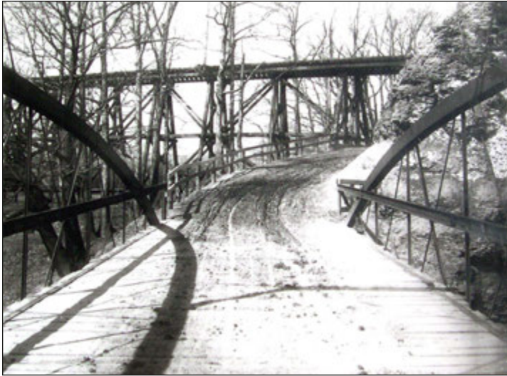
Center section of Days Dam bridge (~1910) over the Black River showing the roadway passing under the Avon Beach & Southern electric railway trestle (courtesy of Black River Historical Society).
