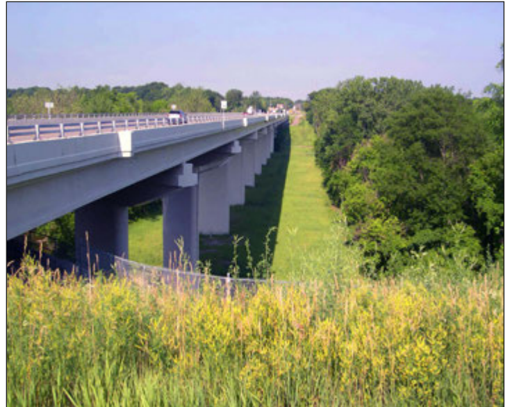
New Garfield Bridge over the Black River as completed in 2003.
