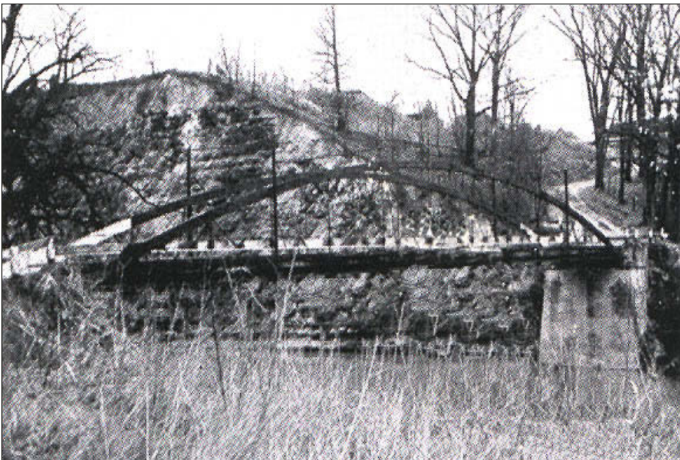
Old North Ridge steel-truss bridge over the Black River in 1908 (courtesy of Ohio Department of Transportation).
