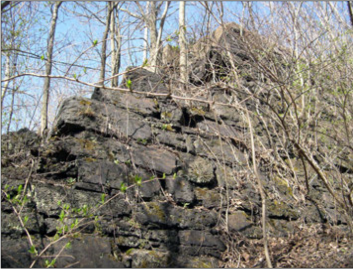
Abandoned causeway's retention wall as it appeared in April 2008.
