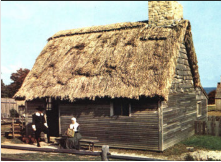
Replica of Elder William Brewster House at Plimoth Plantation. The dwelling was made of clapboard over vertically planked walls with a thatched roof. The Pilgrims called their first settlement Plimoth Plantation meaning a new planting.
