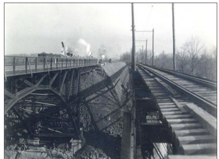
Causeway under construction leading to the steel girders portion of the first East 31 st Street Bridge in 1913. Photograph taken from Avon Beach & Southern electric railway trestle, built in 1905, toward the east. Note impressive stonework for the causeway's retention wall (courtesy of Black River Historical Society).
