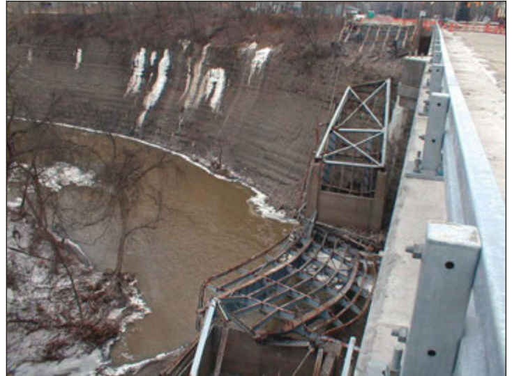
The original Garfield Bridge being demolished by blasting in January 2003.
