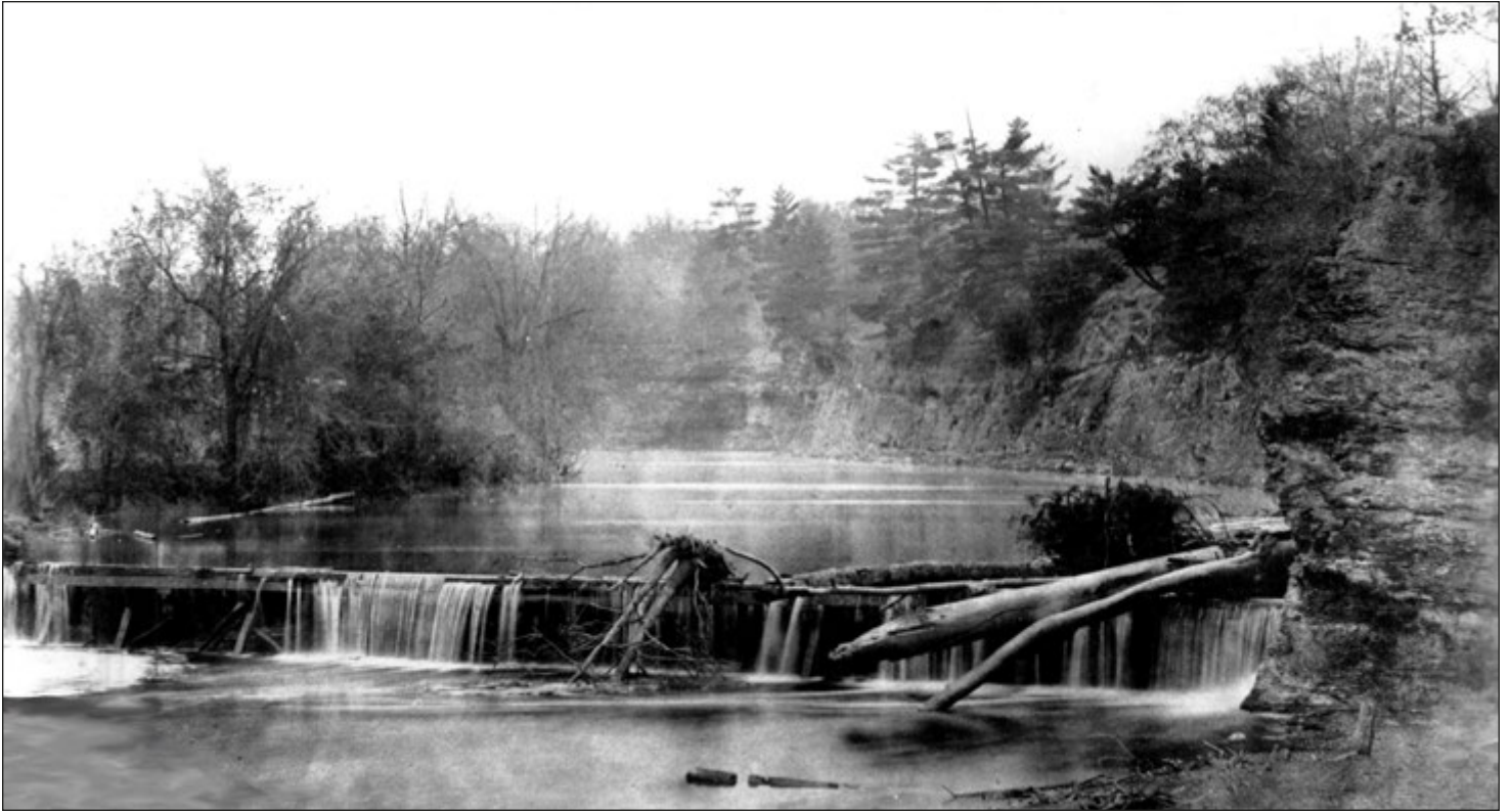
Day's Dam on the Black River; once located upstream of Day's mills to provide a constant head of water for operating the waterwheels (courtesy of Lorain County Historical Society).
