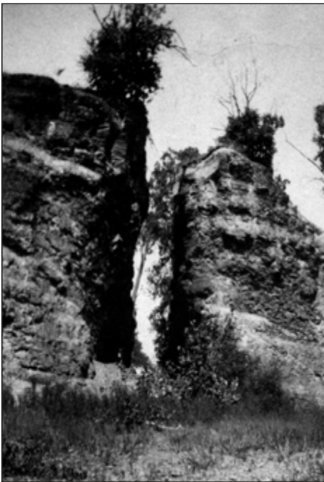
Tunnel cut in the shale bank of the Black River to form a raceway to conduct river water from behind the dam to the waterwheels at the mills (courtesy of Lorain County Historical Society).
