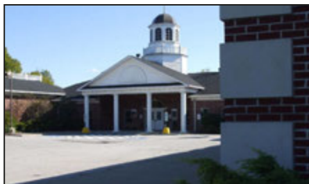
Sheffield's Municipal Complex, 4340 Colorado Avenue, originally built in 1957 as a fire and police station, enlarged in 1999 to house the mayor's office and Village council chambers.
