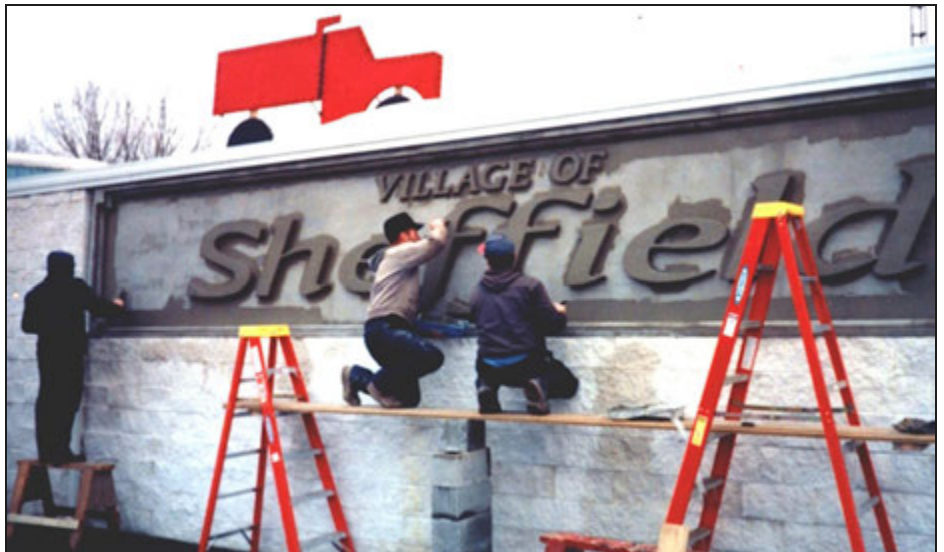
Bill Sheets, Rudy Ackerman, and John Ackerman (left to right) applying the final coat of stucco to the sign.
