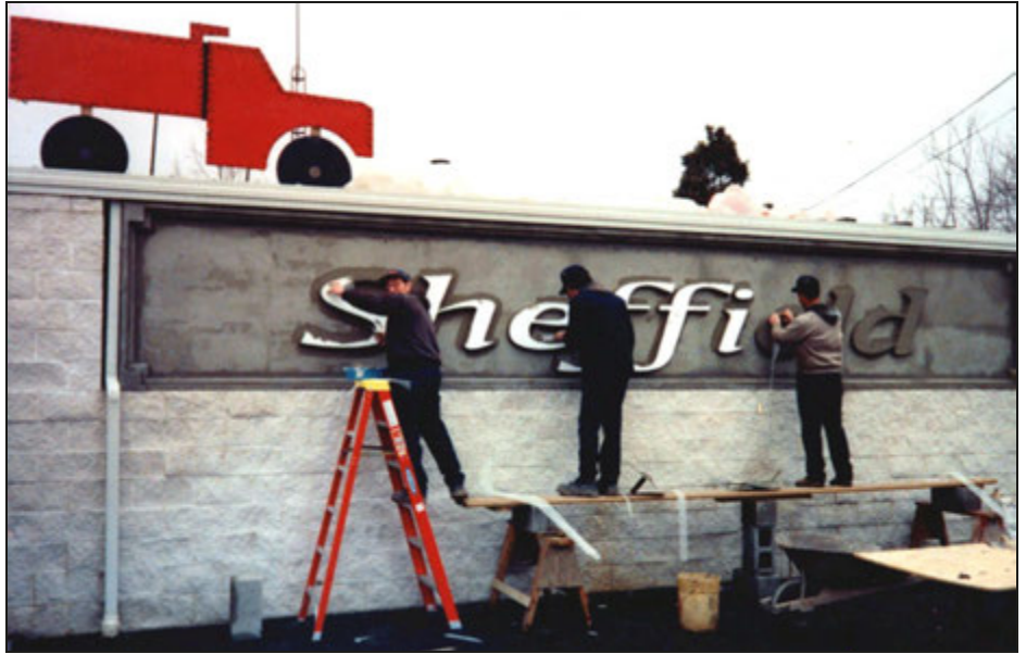
John Ackerman, Larry Sheets, and Rudy Ackerman (left to right) attaching the sign letters on the Village Service Building and starting to coat them with stucco.
