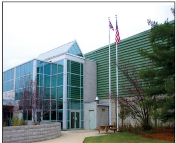
Processing building at the Recovery Complex.
