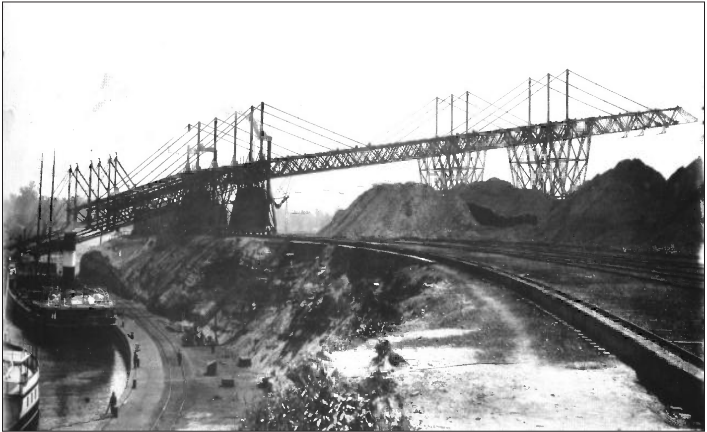
McMyler hoist ore unloader at the steel mill dock on the Black River (courtesy of the Black River Historical Society).
