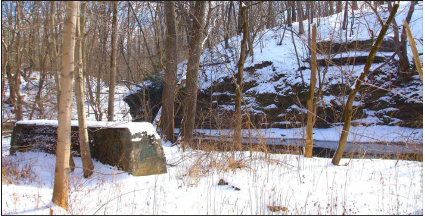
Foundation abutments for the Lake Erie & Pittsburgh Railroad trestle over French Creek in 2011 at the French Creek Reservation.
