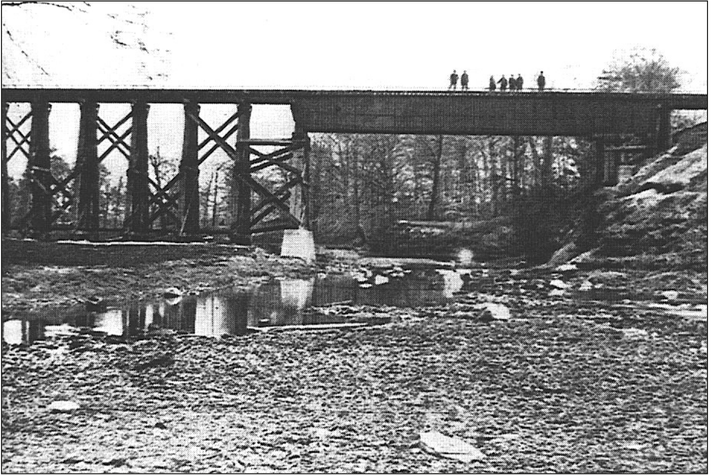
Lake Erie & Pittsburgh Railroad trestle over French Creek on the James Day farm in April 1917 (courtesy of Lorain County Metro Parks).
