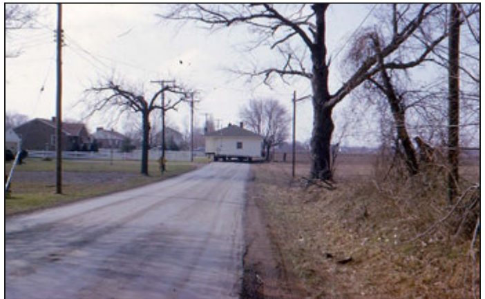
Chuck Gubeno's house at southwest corner of intersection being moved farther south on Abbe Road when Detroit Road was widened. This house was later torn down to make way for the Cobblestone shopping area.
