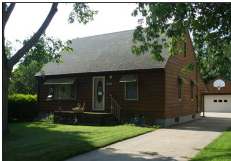
Current photograph of the Klingshirn house at 4531 Day Street.
