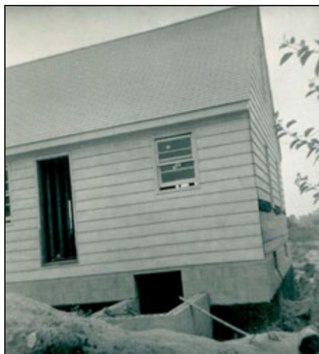
Construction of Butch and Elaine Klingshirn’s home at 4531 Day Street in 1956. Butch (right) and his brother Dub are shown attaching siding. The cellarway in the second view did not pass a code inspection because it was too close to the septic tank and had to be abandoned. The third view shows the house nearing completion in October 1956 (courtesy of Bruce and Sue [Klingshirn] DiVaccaro).
