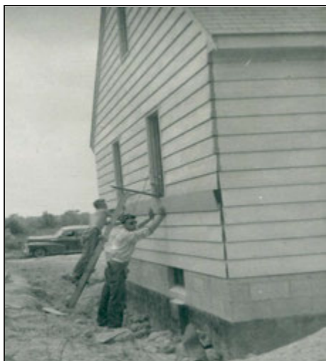
Construction of Butch and Elaine Klingshirn’s home at 4531 Day Street in 1956. Butch (right) and his brother Dub are shown attaching siding. The cellarway in the second view did not pass a code inspection because it was too close to the septic tank and had to be abandoned. The third view shows the house nearing completion in October 1956 (courtesy of Bruce and Sue [Klingshirn] DiVaccaro).
