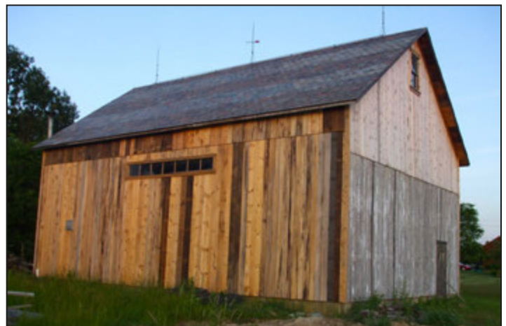
Rear view of the restored Daniel Garfield Barn in Avon.
