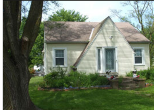
Wharton House, 4507 Day Street—a Sears house, The Claremont , was built by John Wharton ~1925.
