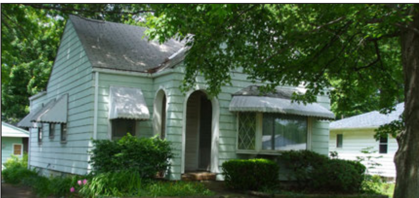
King House, 4587 French Creek Road, a Sears house— The Berwyn , was built by Maxwell and Helen (Day) King ~1935.
