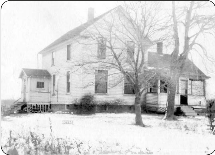
Edward Karney House, 1515 Lake Breeze Road in Sheffield Village, was originally constructed in the Greek Revival Style before 1857. This 1943 photograph illustrates the primary features of this style that was popular for farmhouses during the period 1825-1860, such as a wide cornice board and partial return of the eaves across the gable front (courtesy of James and Joyce Toth).
