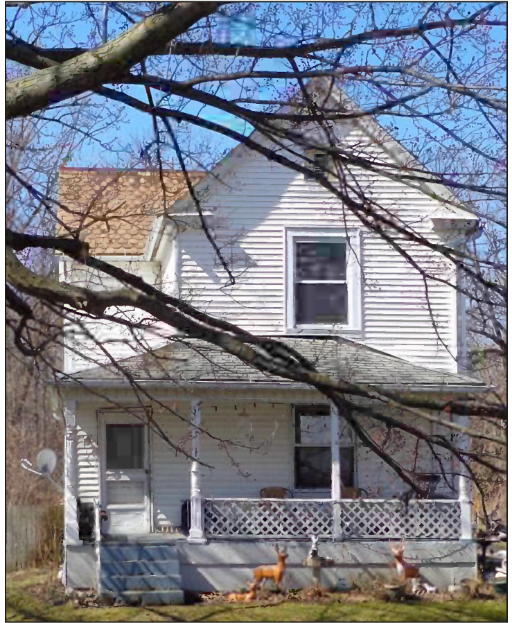
John Fox House, 998 Lake Breeze Road in Sheffield Lake, was built circa 1840s in the Greek Revival Style. John Fox owned and farmed land on both sides of Lake Breeze Road for nearly 40 years. The house is believed to be the oldest homestead still in existence on Lake Breeze Road.
