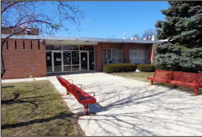
The William W. Barr Elementary School, at 2180 Lake Breeze Road, was built in 1961 and named in honor of a long-time superintendent of the Sheffield-Sheffield Lake City School District.
