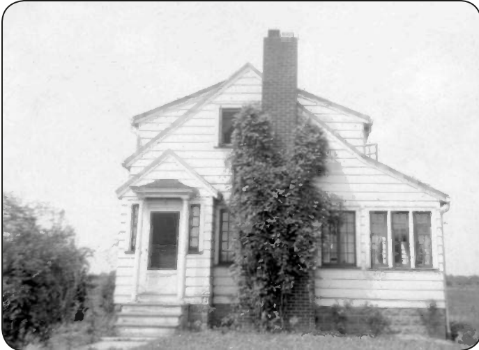
Gawn-Cotton House, at 882 Lake Breeze Road, was built in the Folk Vernacular Style circa 1910. The house originally had a set of Doric-style columns at the sides of the front entrance as shown in this 1939 photograph.
