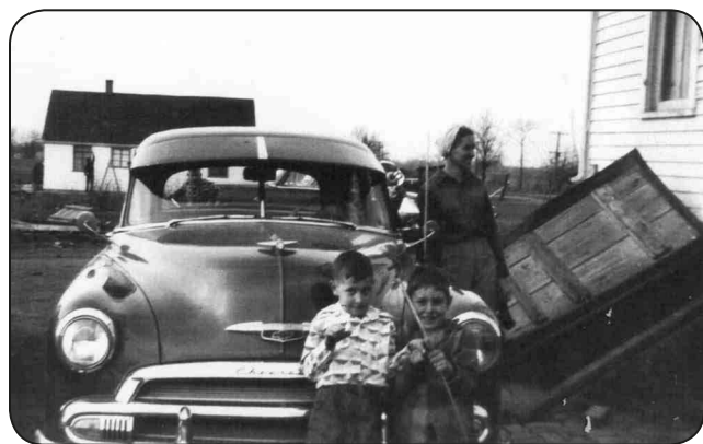
View of the back side of the Thomas Fox House in the early 1950s with the Pratt family and their new Chevrolet automobile. Note the exterior basement doorway (courtesy of Christine [Pratt] Neuber).
