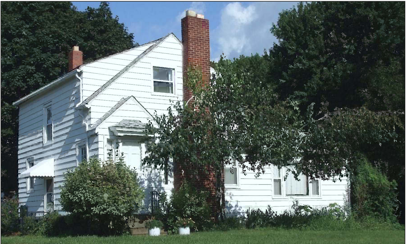
The front-gable façade of the Gawn-Cotton House is dominated by a massive chimney that facilitates a large fireplace. This recent photograph shows that an extended side wing and a picture window have been added to the original design.
