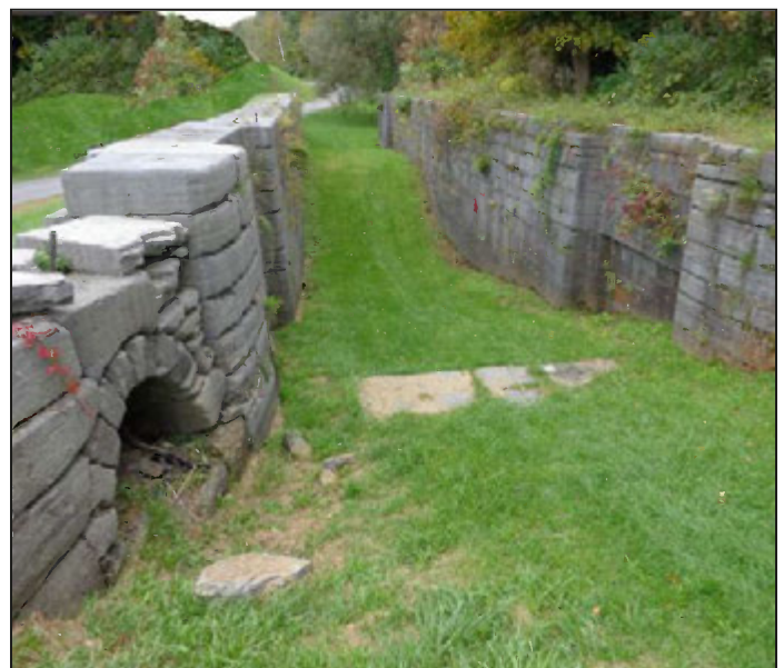
Remains of the canal and locks at Little Falls, New York, which were used by boats to bypass the rapids on the Mohawk River in the early 1800s.
